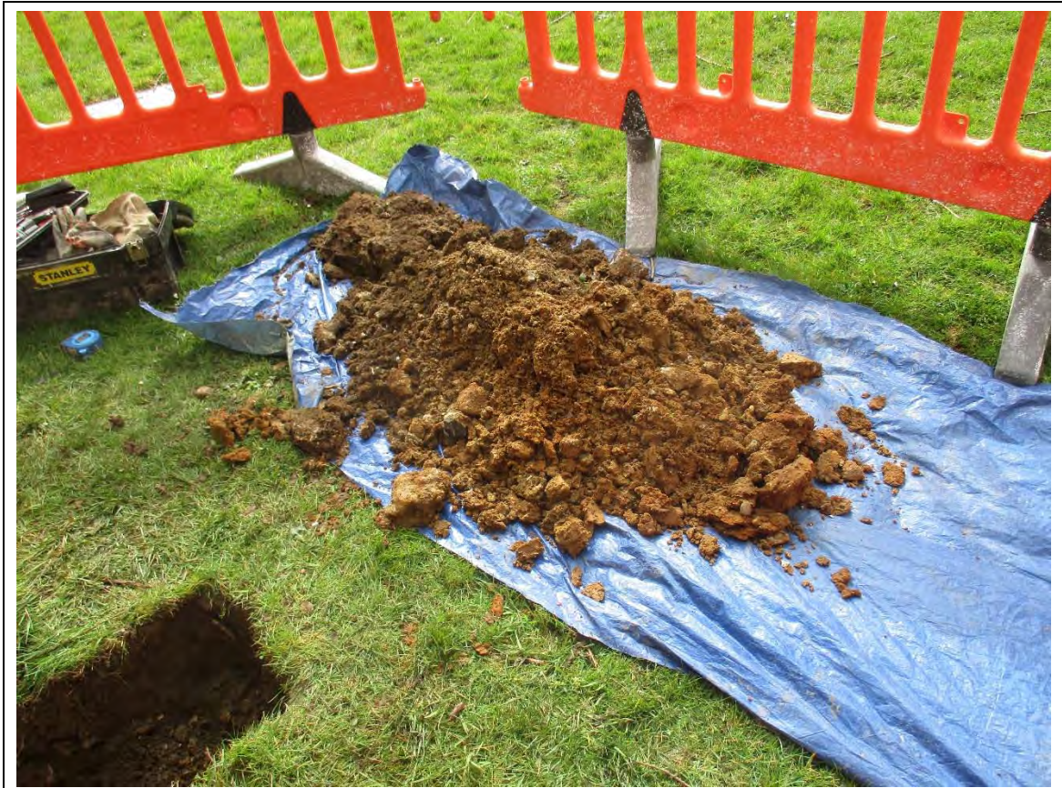
Inspection pit: IP03 spoil
