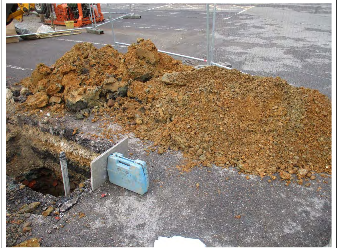
Trial pit: TP02 spoil
