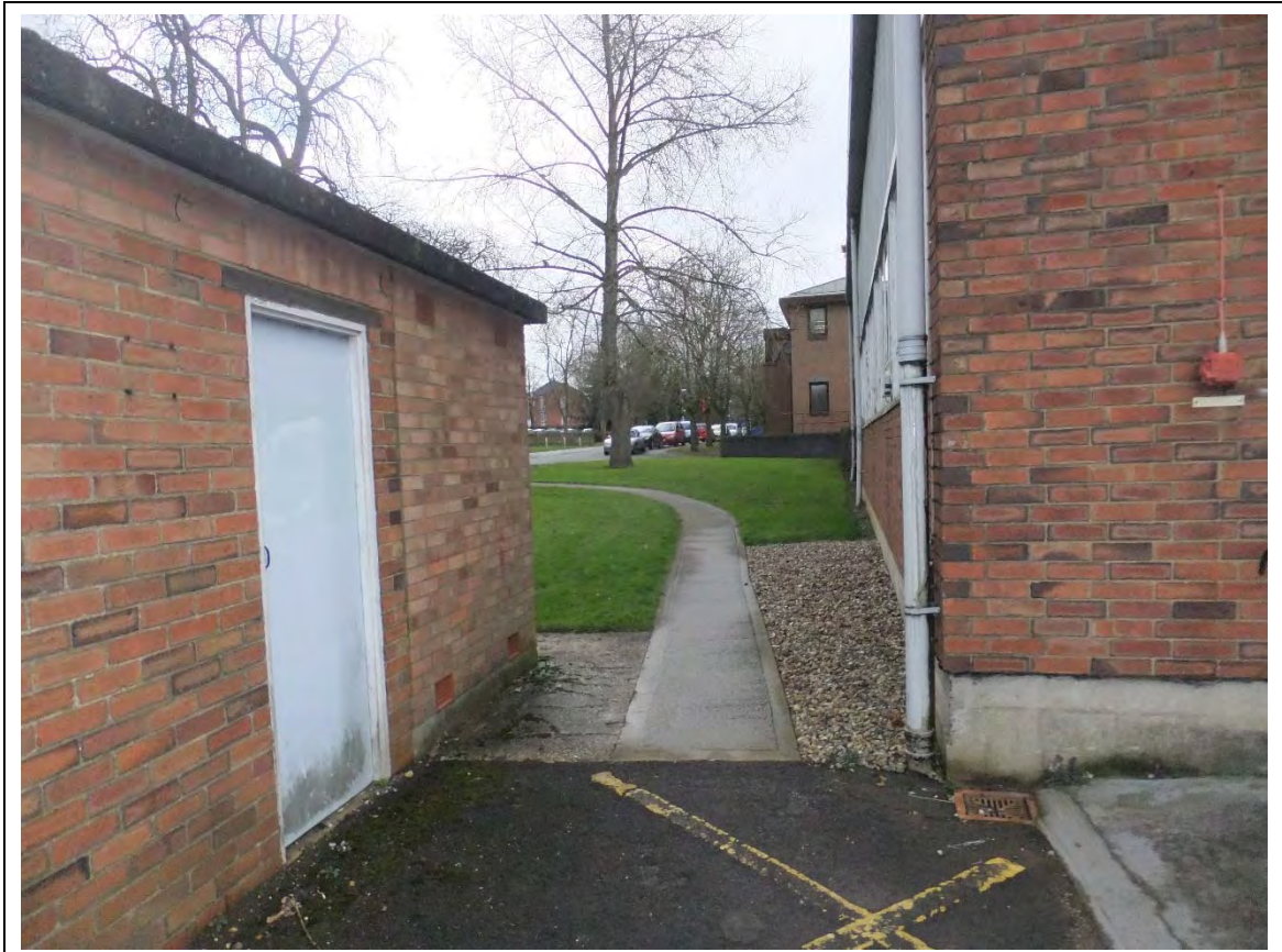
View looking west along the southern elevation of the Engineering Building
