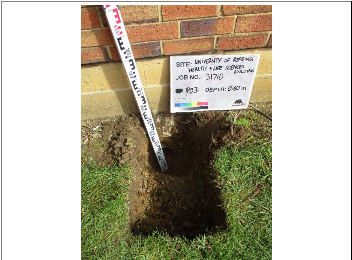
Inspection pit: IP03 profile
