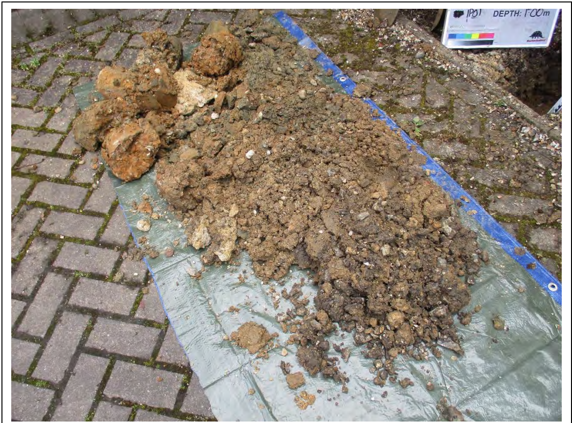
Inspection pit: IP01 spoil
