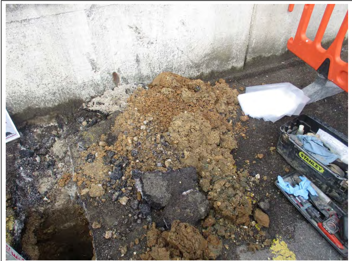
Inspection pit: IP02 spoil
