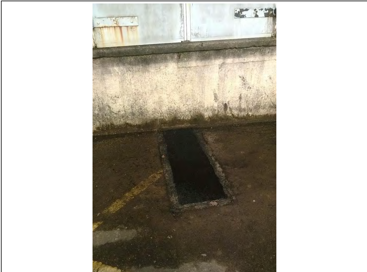
Inspection pit: IP02 reinstatement
