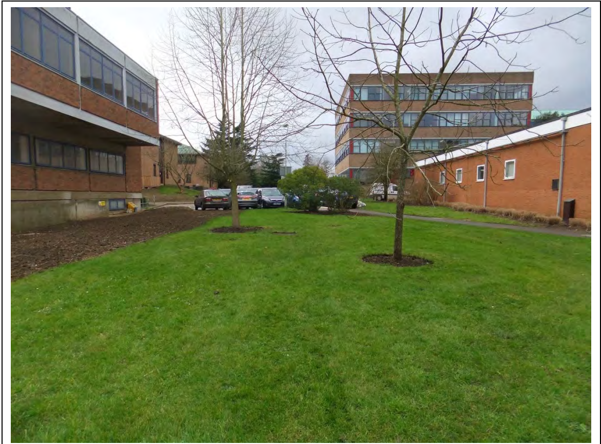
View looking west along the northern elevation of the Engineering Building
