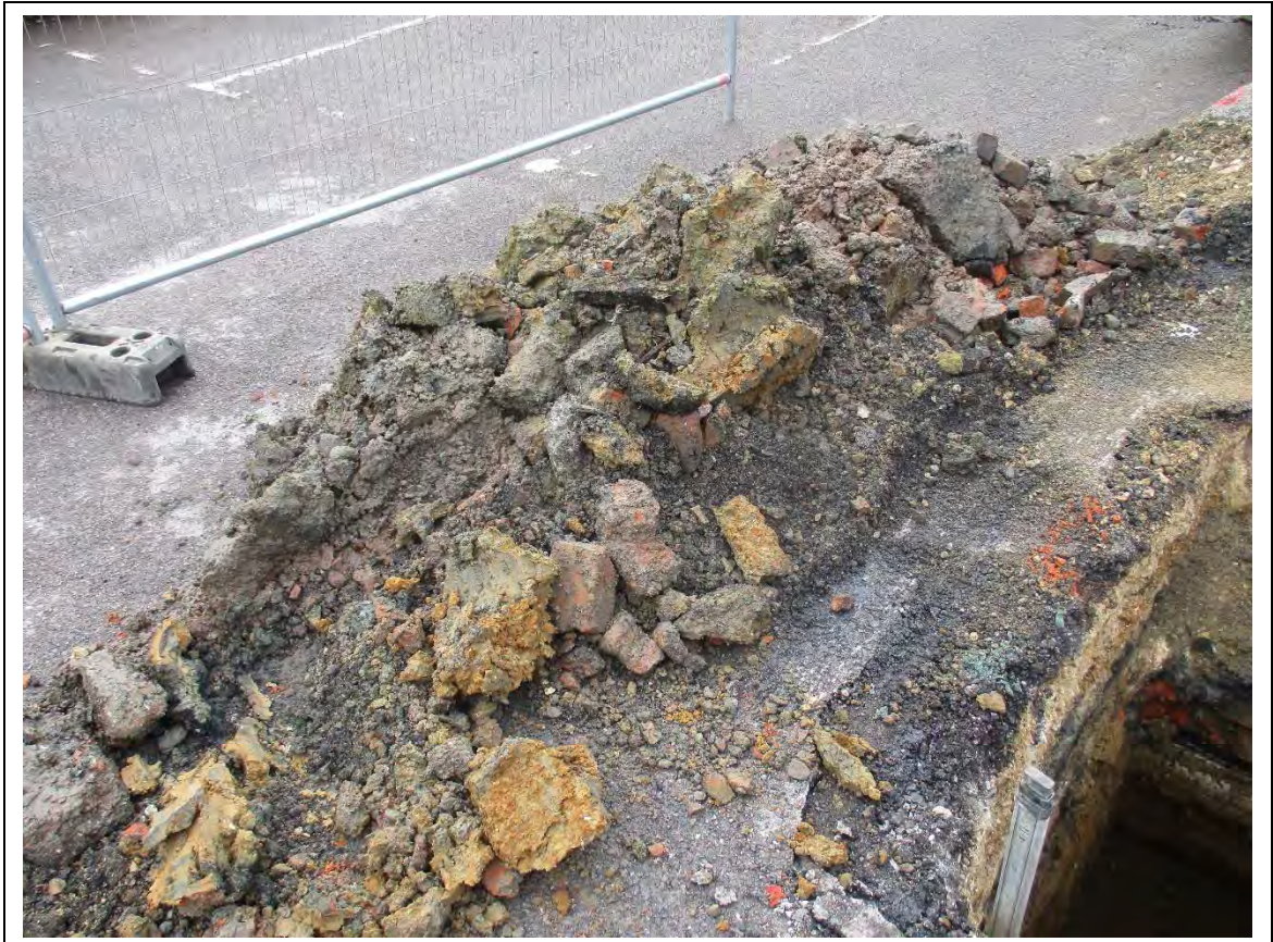
Trial pit: TP02 spoil
