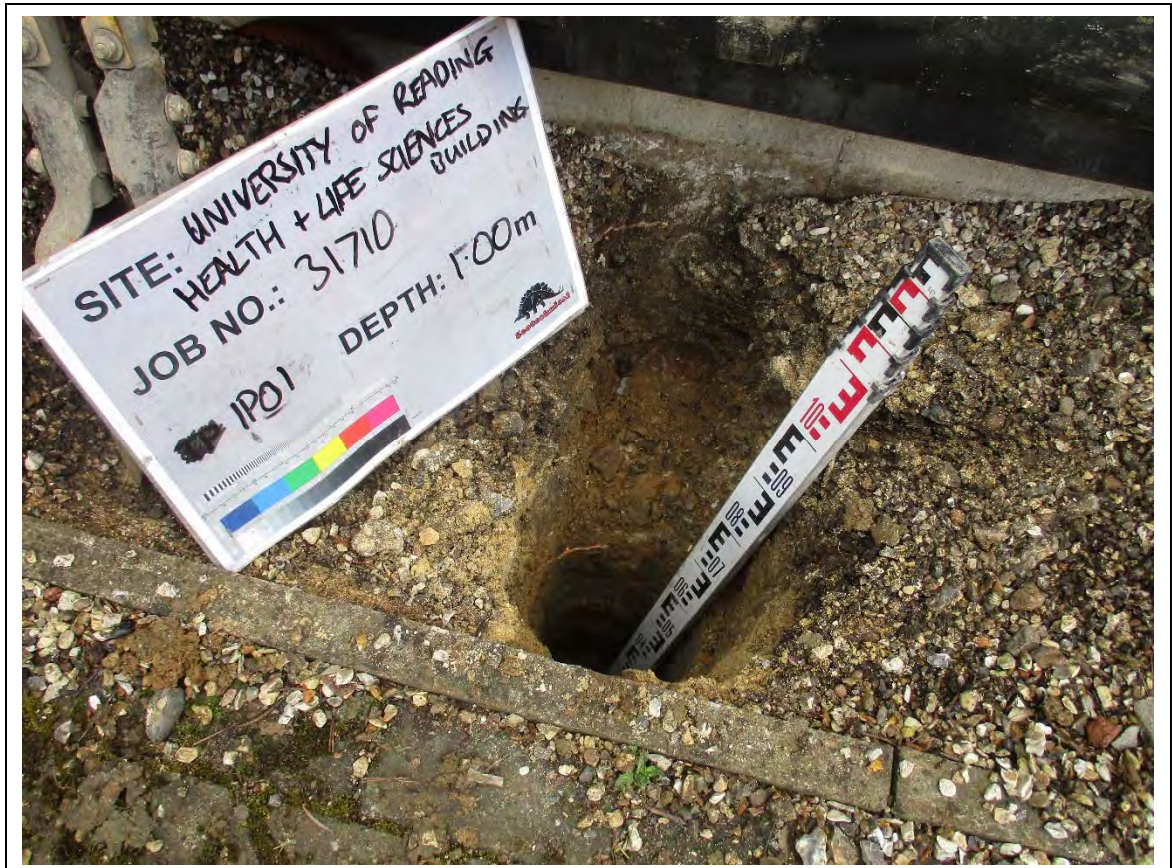
Inspection pit: IP01
