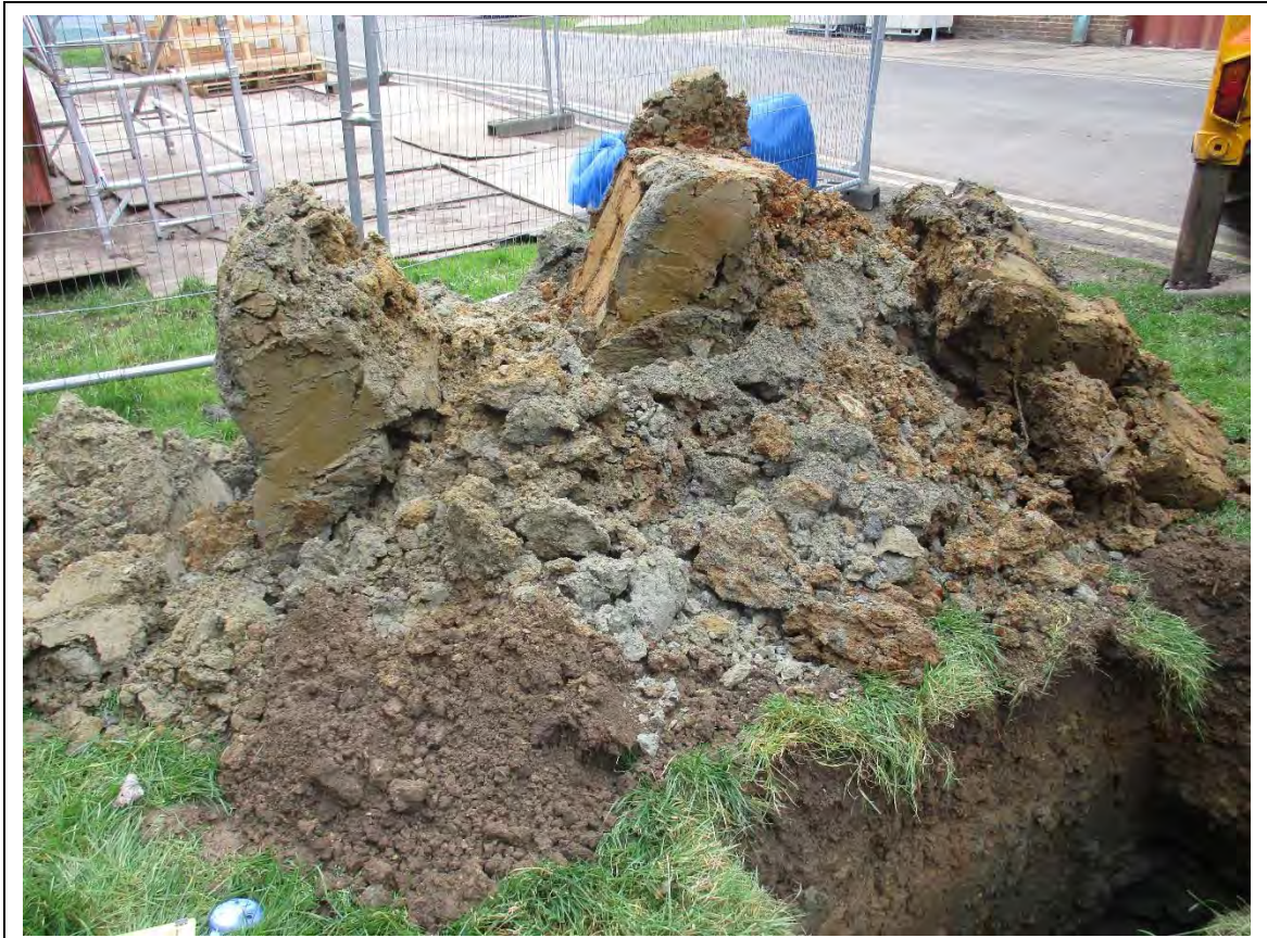
Trial pit: TP03 spoil
