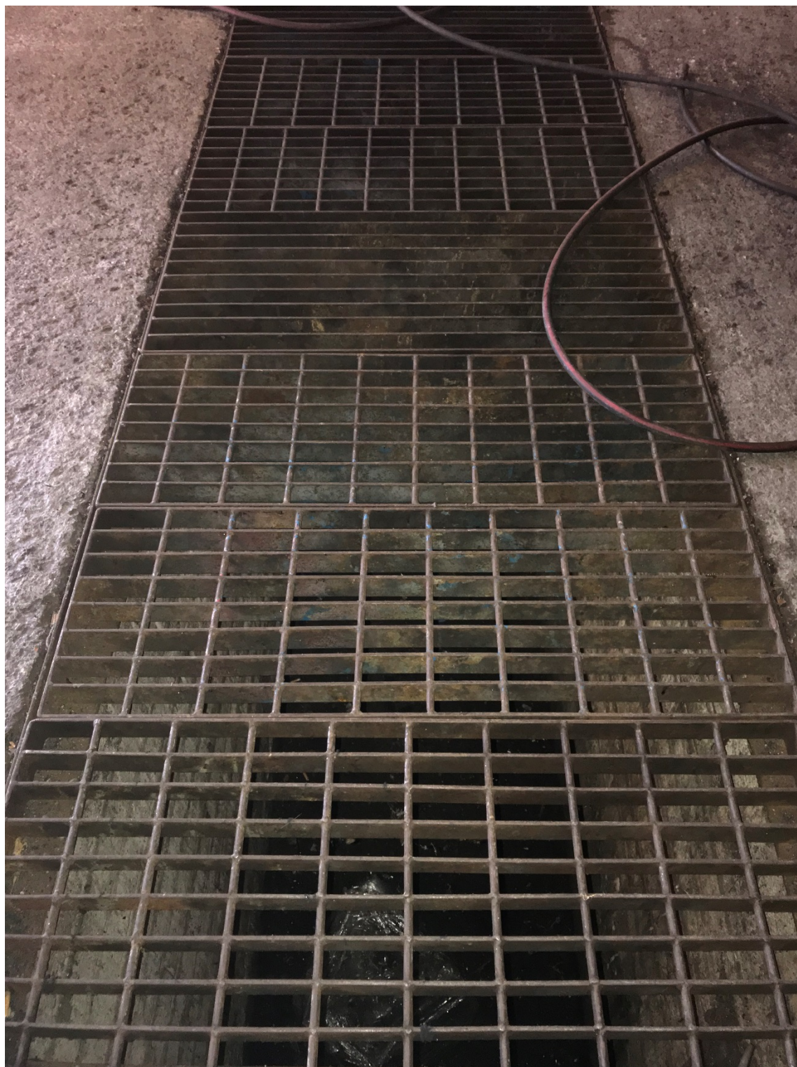
Inspection pit within tyre fitters
