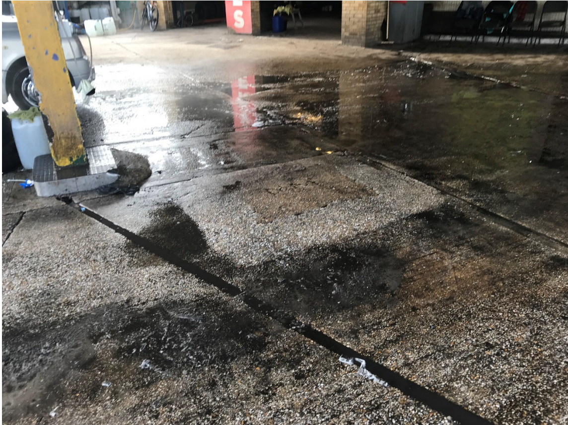
Concrete 'mound' denoting suspected location of former fuel tank cover
