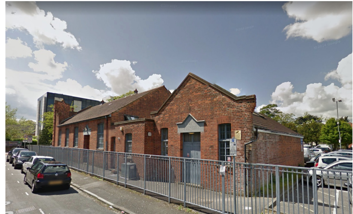
External looking South from Kingsgate
