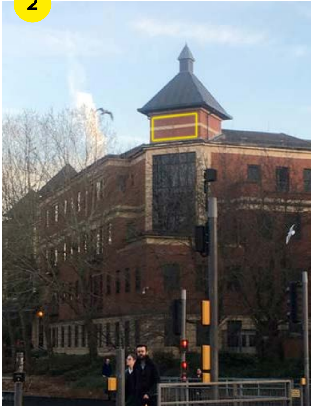
Brick Area at top of No.1 New Century Place
