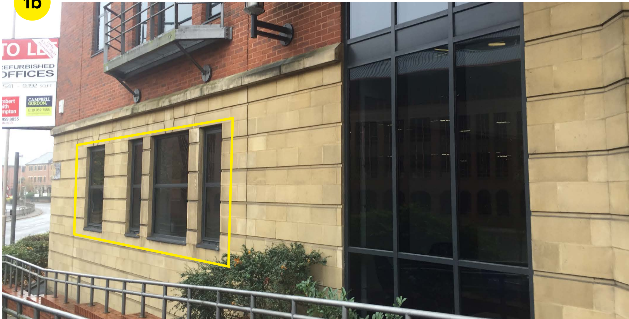
Windows on ground floor (1b) of No.2 New Century Place
