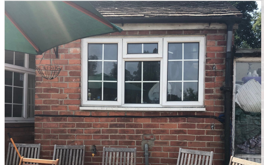
Existing kitchen extension
