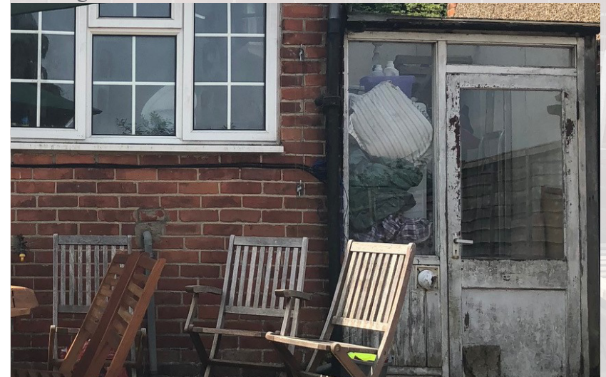
Existing Lean-to extension
