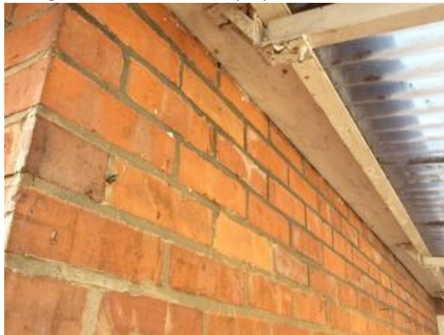
Figure 4. The well fitting wooden soffits and edging around the tops of the wall of the south facing aspect of the bungalow.
