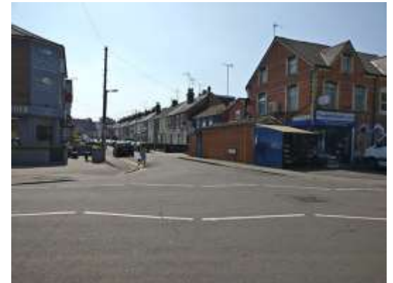
Side extension at Punjab Stores built up to the pavement boundary
