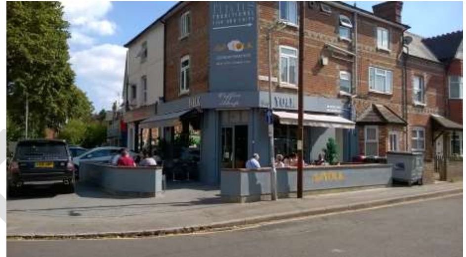
Existing external dining area
