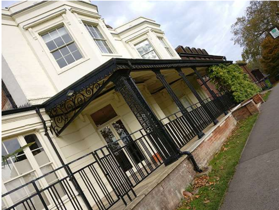
Victorian wrought iron canopy
