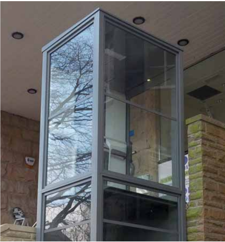
Glazed shaft and upper floor level entry
