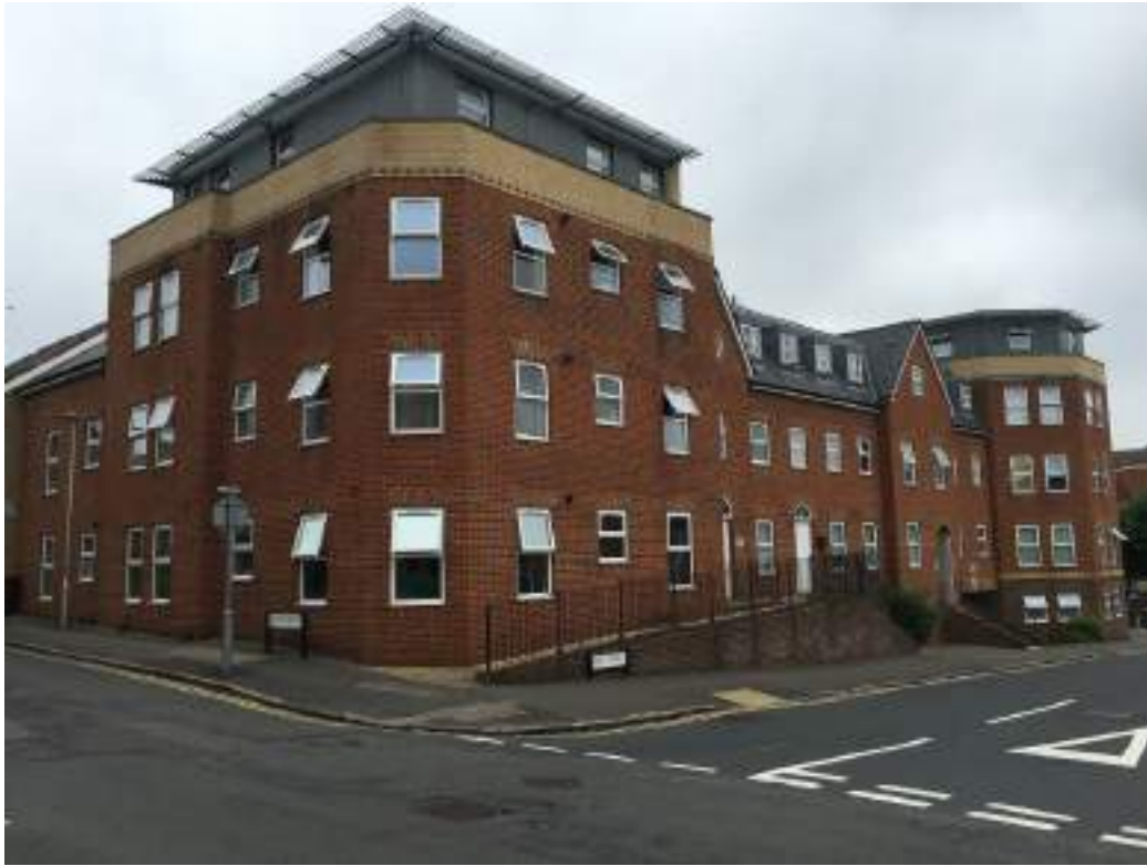
Figure 18 Corner of East View Place at South Street
