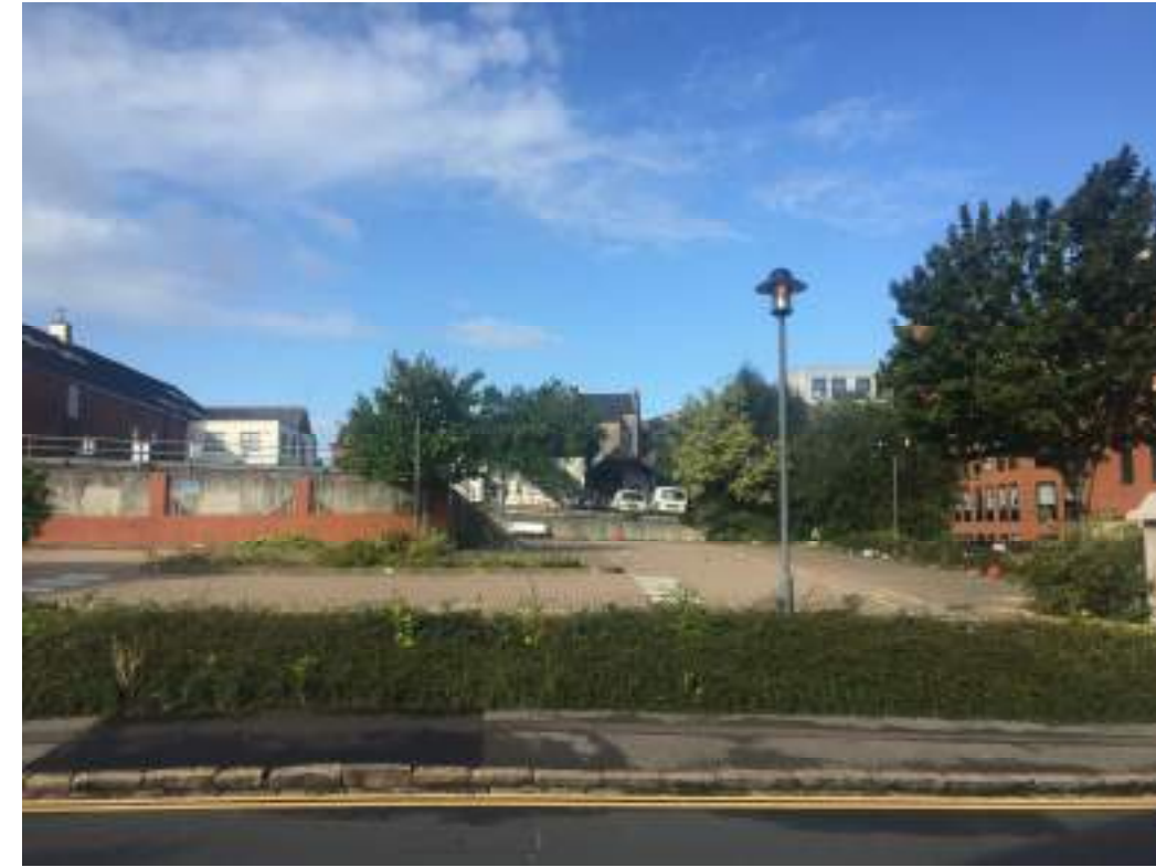
Figure 06 View of retaining walls along site boundary
