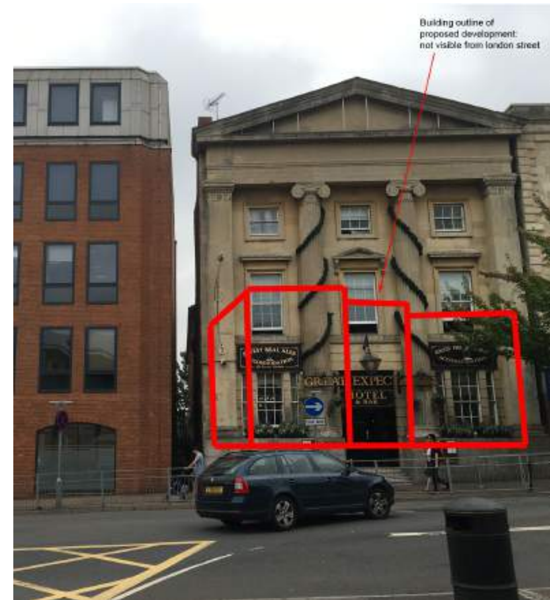
Figure 40 Visual Impact study – view from London Street looking east
