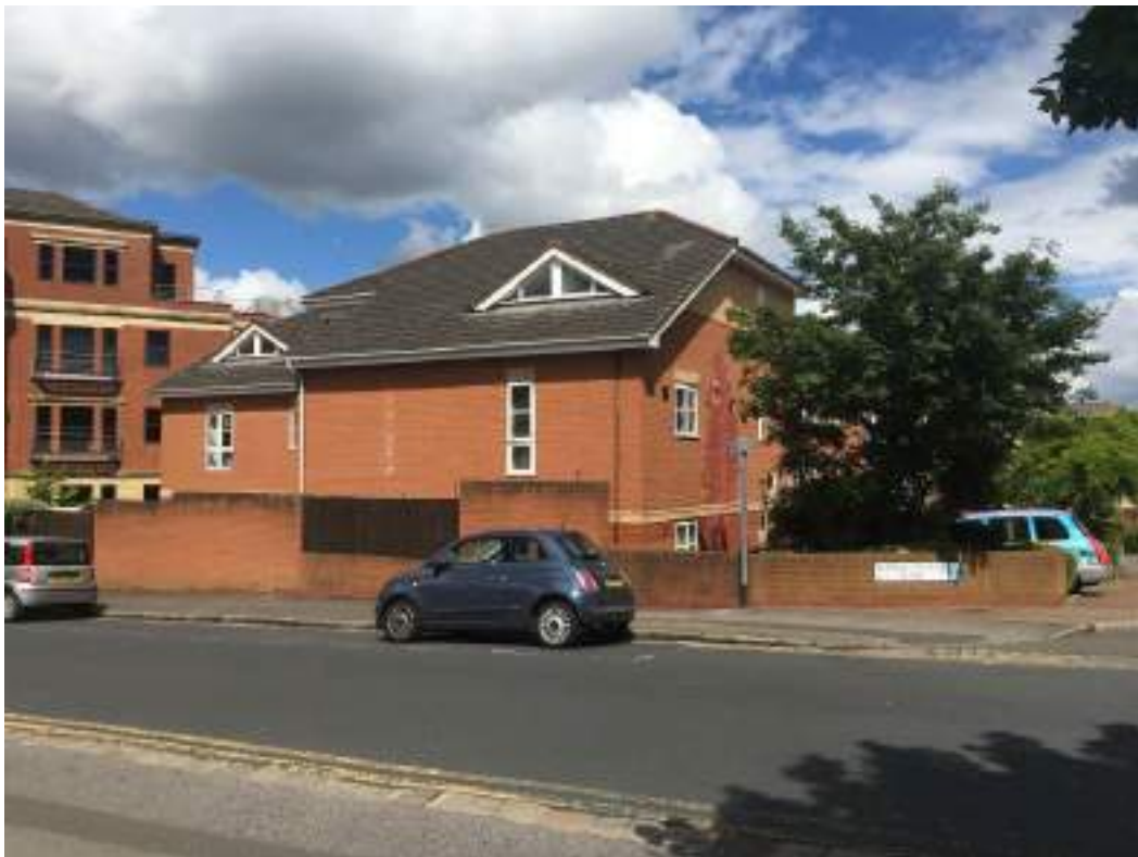
Figure 15 Gable of Bourne-Stevens Close facing site
