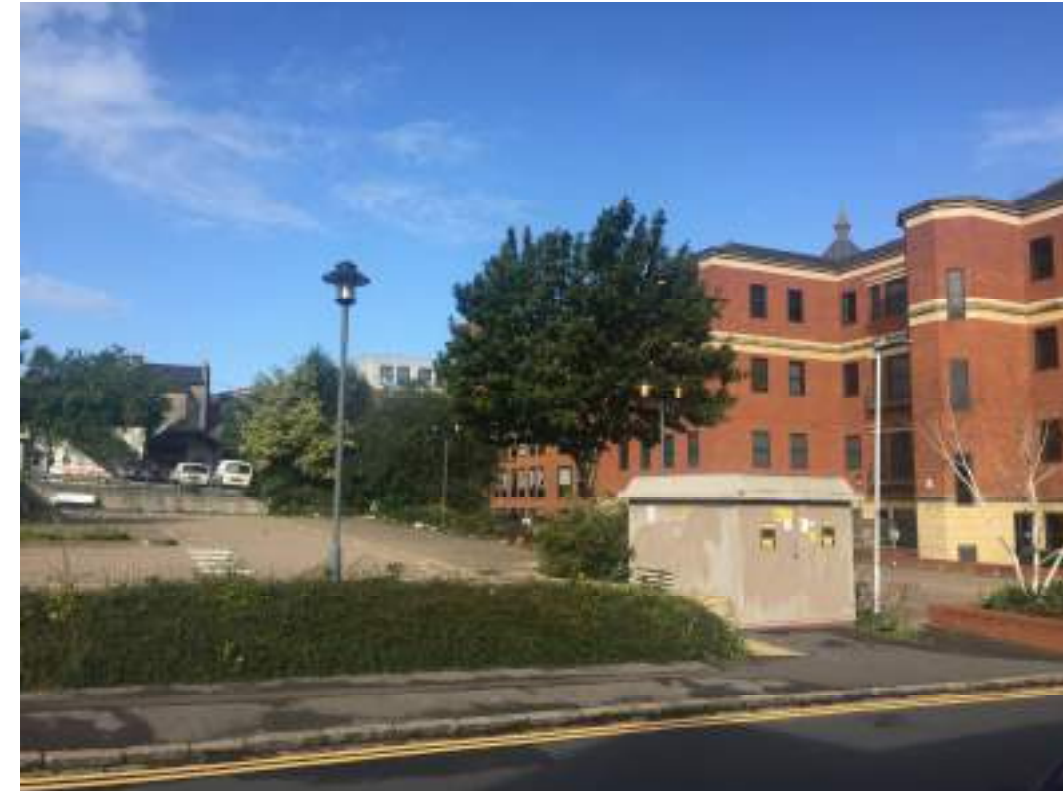
Figure 09 View of the existing substation from within the site
