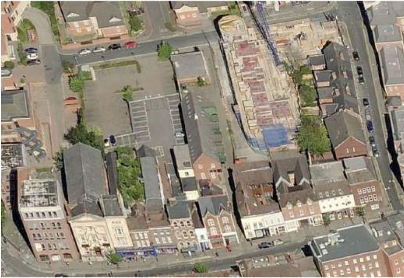
Figure 23 Aerial view – from west over London Street
