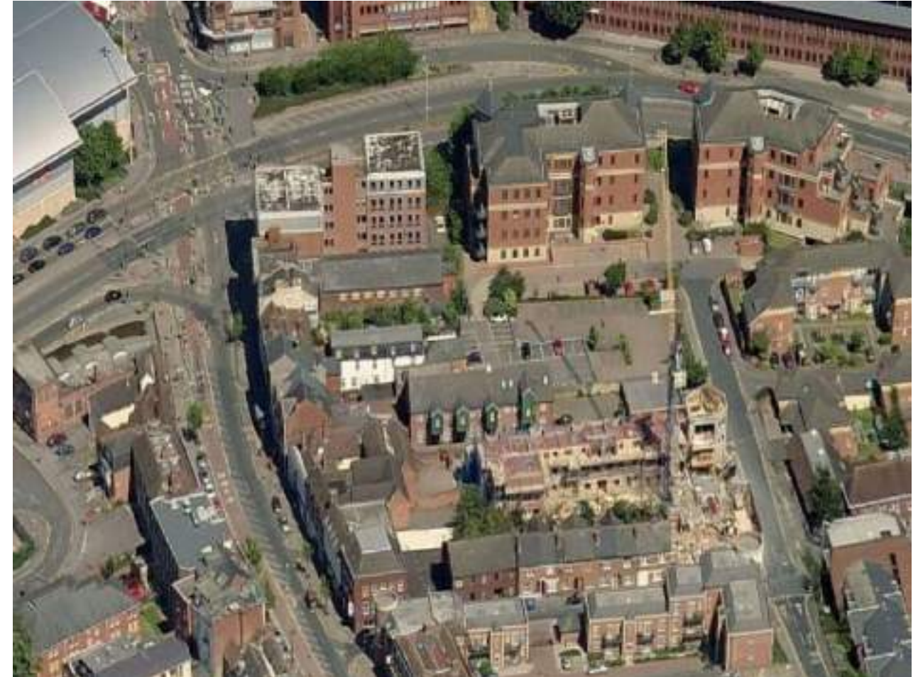
Figure 24 Aerial view – from south to Queen's Road
