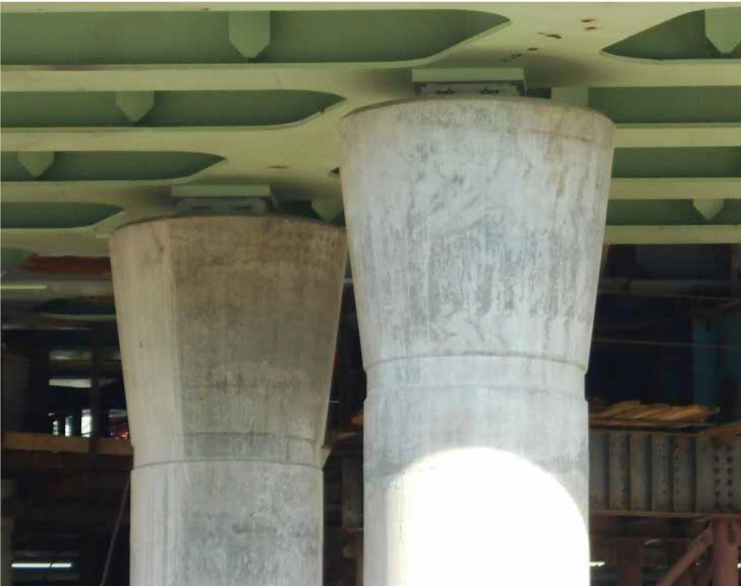
Figure 82. Example of tapered column head
