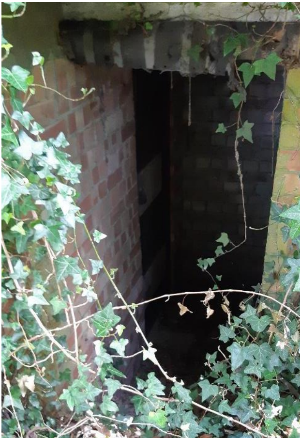
Photograph 11. The doorway to the underground air-raid shelter.
