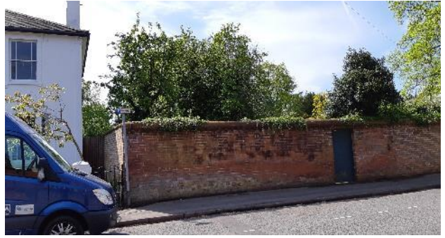
Photograph 8. A brick wall boundary along Upper Redlands Road.
