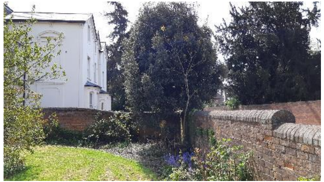
Photograph 10. Boundary brick wall along Redlands Road.
