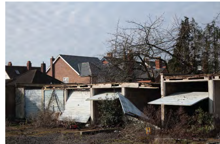
Existing garages (South)
