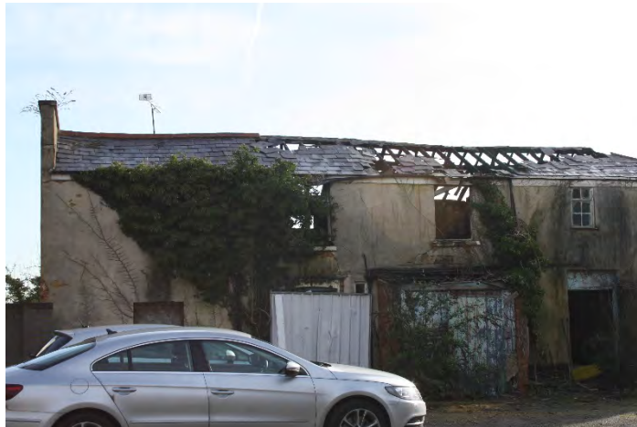
Existing out Buildings (East)
