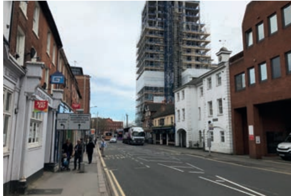
Figure 6.6 Character Area B: Forbury South. View from King' Road, with commercial units lining the street frontage and 120 King's Road in the backdrop.
