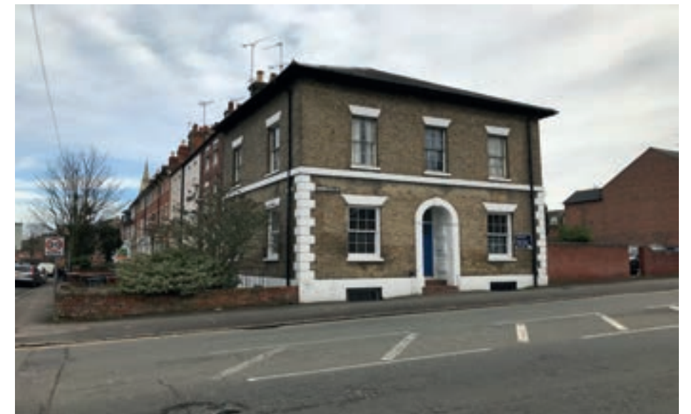
Figure 5.15 No. 9, Sidmouth Street
