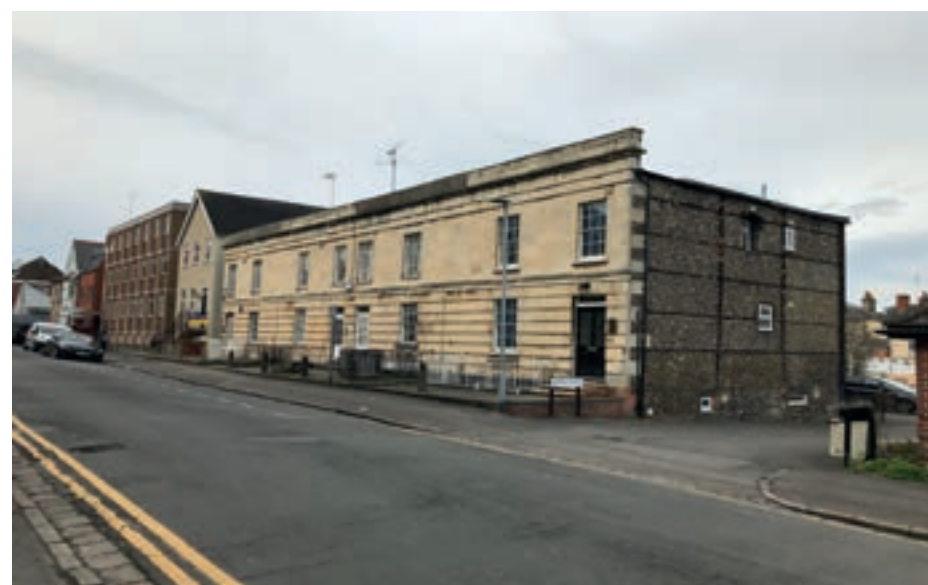
Figure 5.17 Nos. 43–49, South Street
