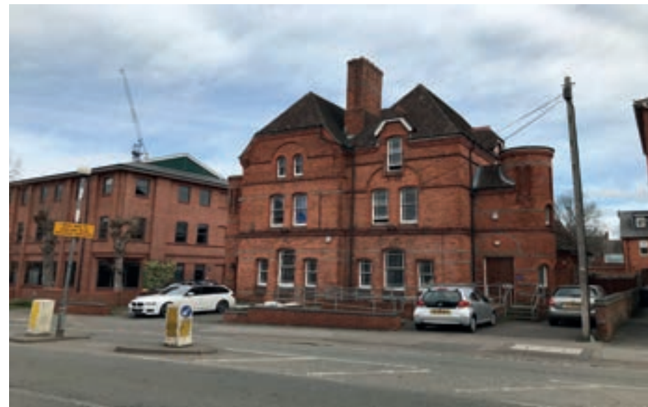
Figure 5.14 Nos. 3 & 5, Sidmouth Street
