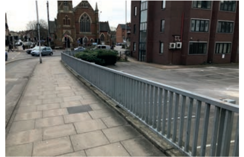
Figure 6.3 Site. View of railings lining east side of Site.
