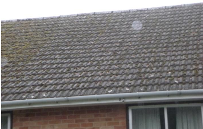
Plate 3. Typical view of the roof tiles
