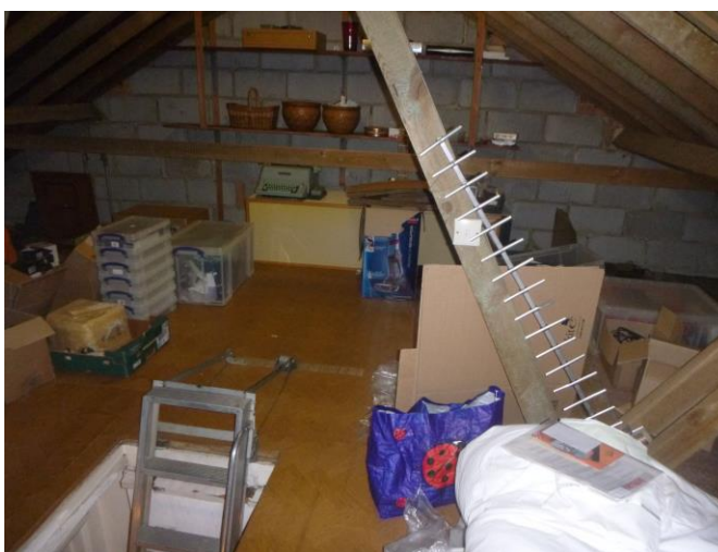
Plate 6. Typical view of the internal void space
