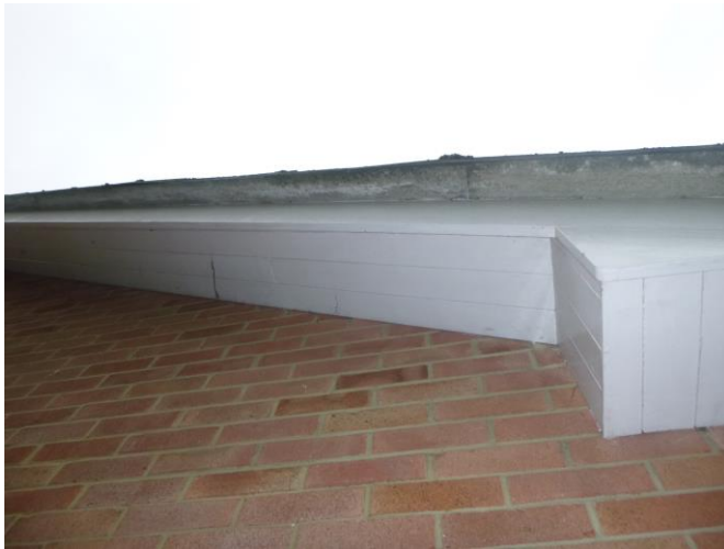
Plate 4. Typical view of the soffit and fascia
