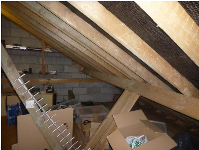
Plate 5. Typical view of the internal void space
