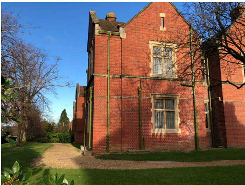
Fig 2- Corner of Redlands Road and Upper Redlands Road Elevation
