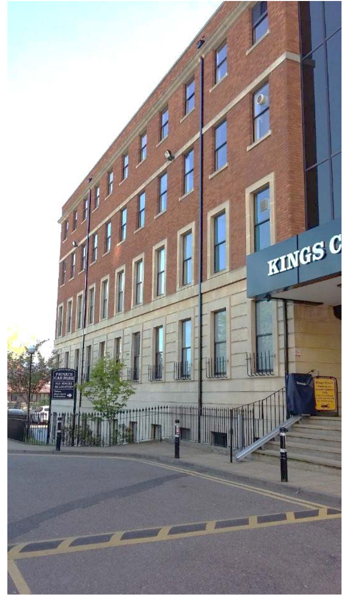
Fig 13. View of 185 Kings Road.
