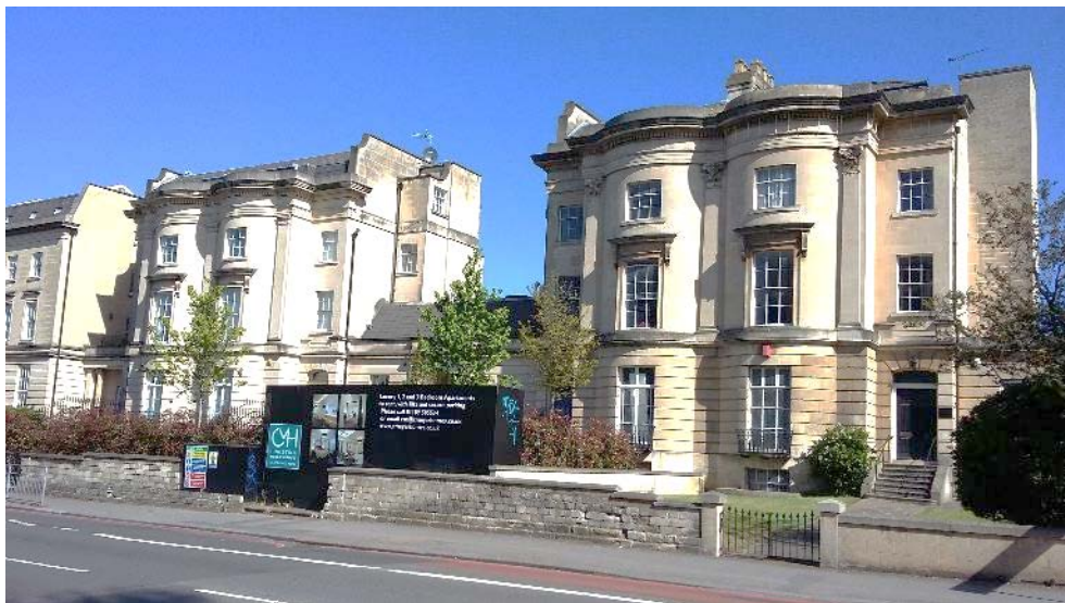
Fig 14. View of 173-179 Kings Road.
