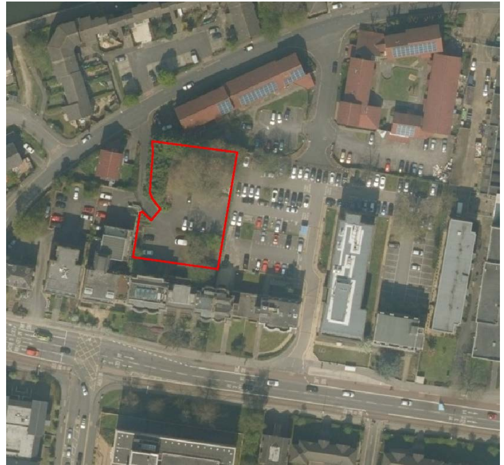
Fig 1. Aerial photograph of the application site.
