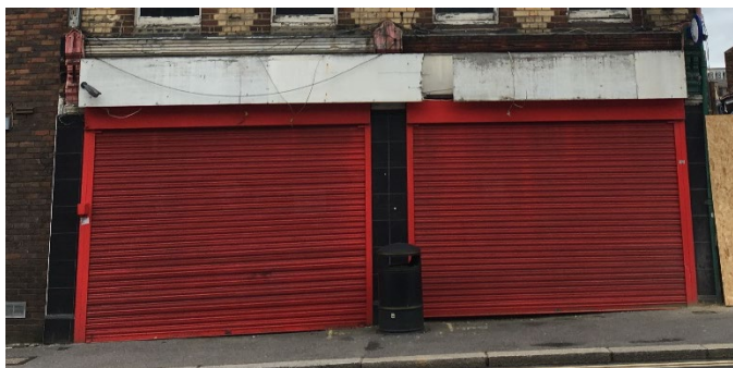
Plate 4: Modern shop front
