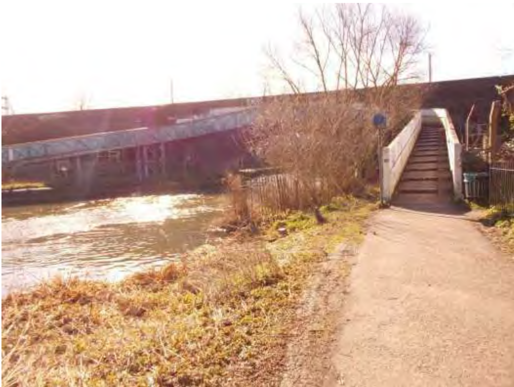
Plate 6: The pedestrian and railway bridge crossing over the River Kennet
