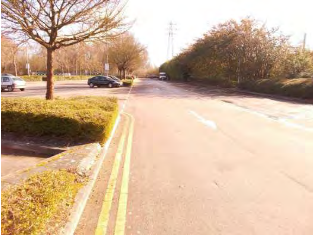
Plate 1: Tesco Superstore car parking and access road
