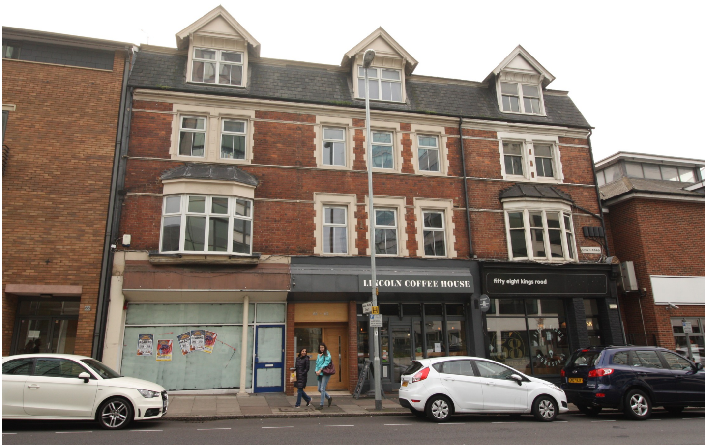
Figure 2: View of front elevation of the existing property (North elevation) taken from Kings Road, 62 is the left hand side unit.
