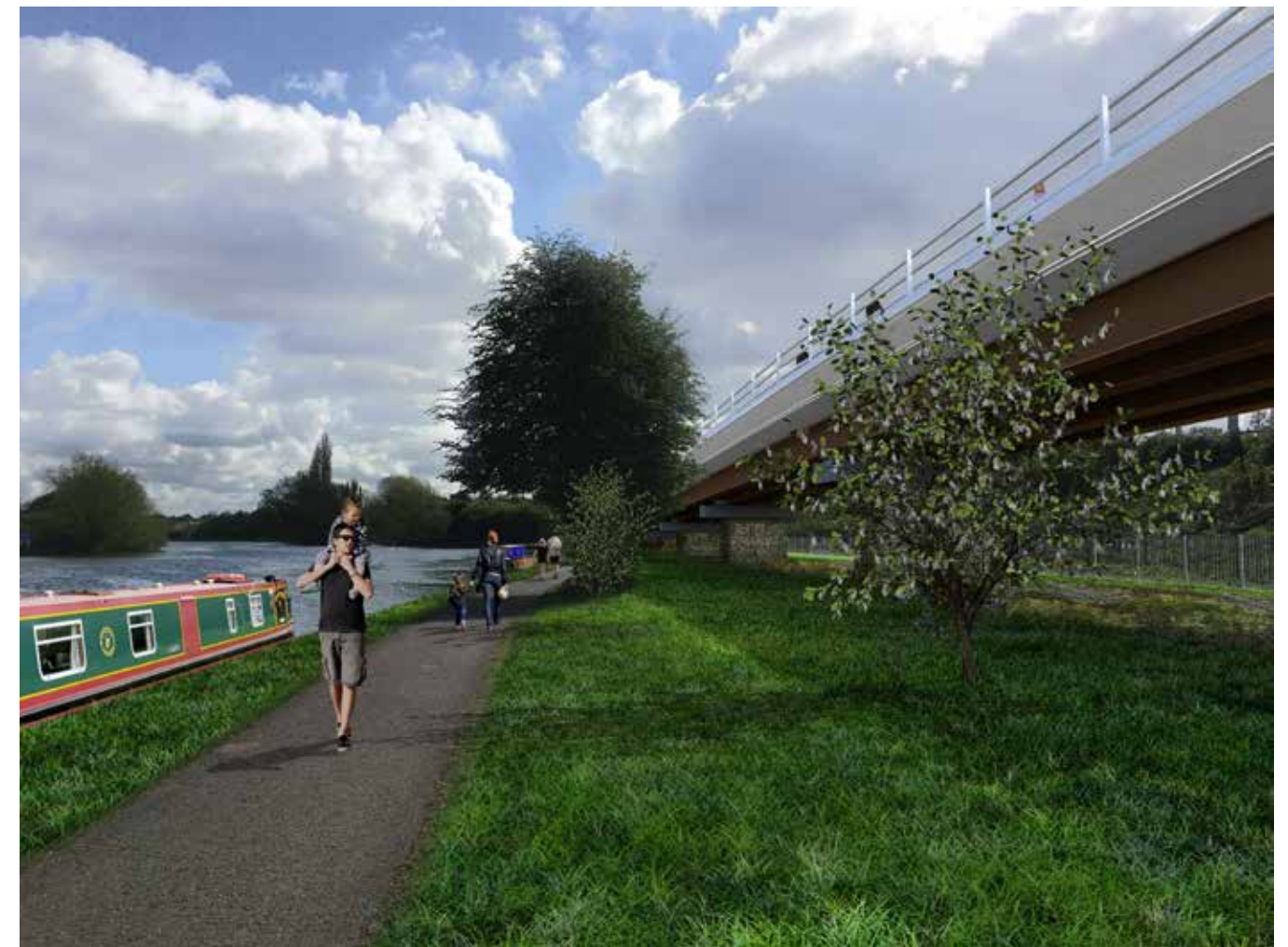
Figure 14. Artist's impression of gabion-clad columns.
