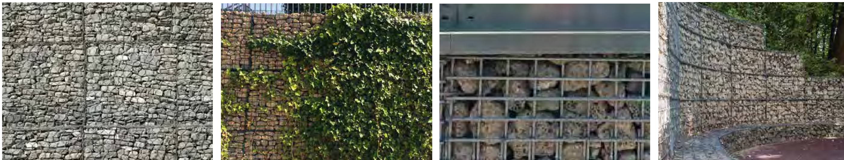
Figure 15. Examples of gabion walls
