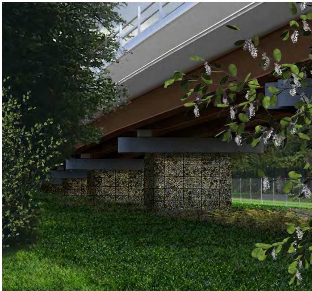
Figure 13. Close-up example of gabion-clad column
