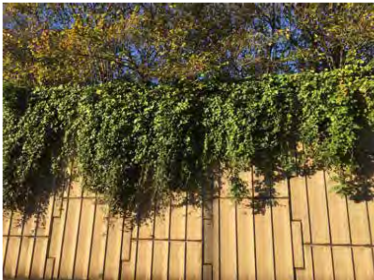
Figure 10. Example of ivy growing over and down a structure
