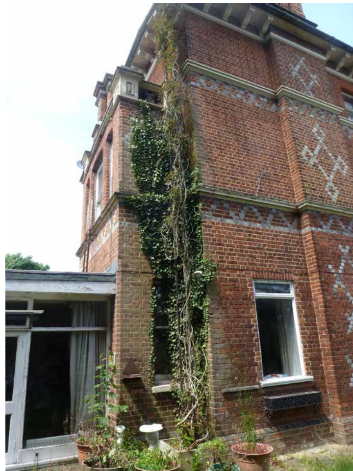
Photo 4: Rear elevation & side extension
