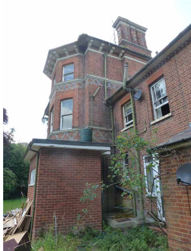
Photo 8: Rear elevation & extension
