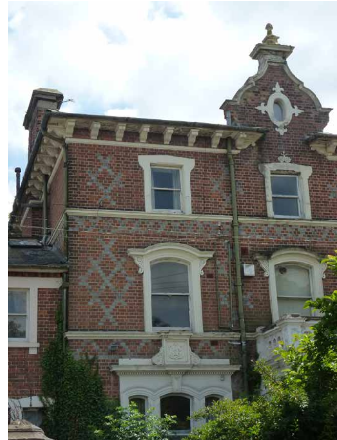
Fig 12: Photograph of existing front elevation detailing
