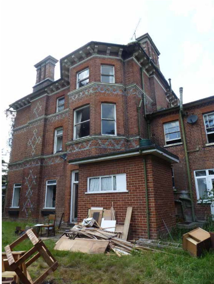
Photo 7: Rear elevation & extension
