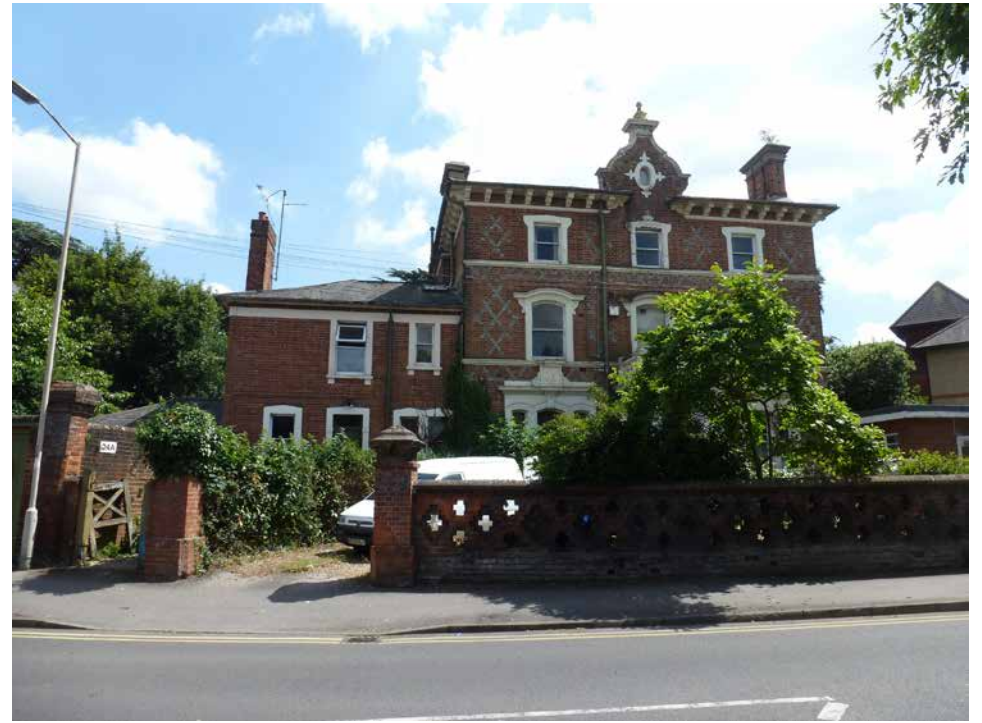
Photo 20: Front view from Southcote Road
