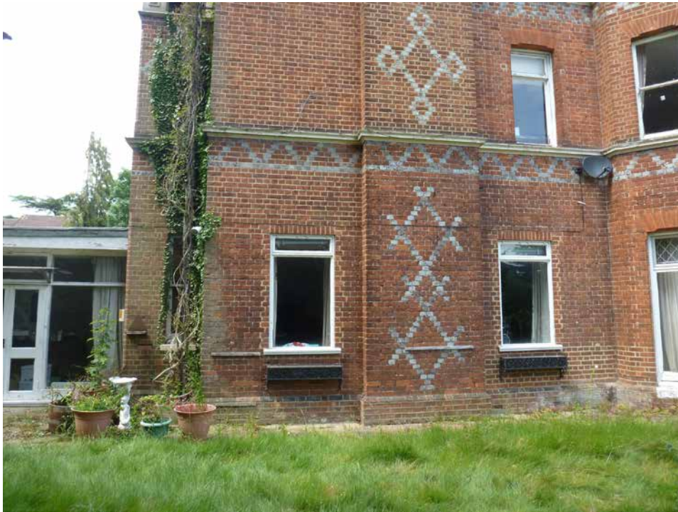
Photo 5: Rear elevation & side extension
