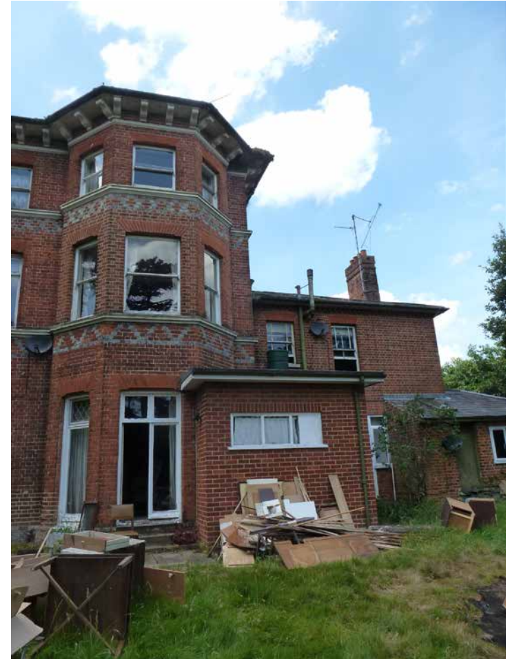
Photo 6: Rear elevation & extension
