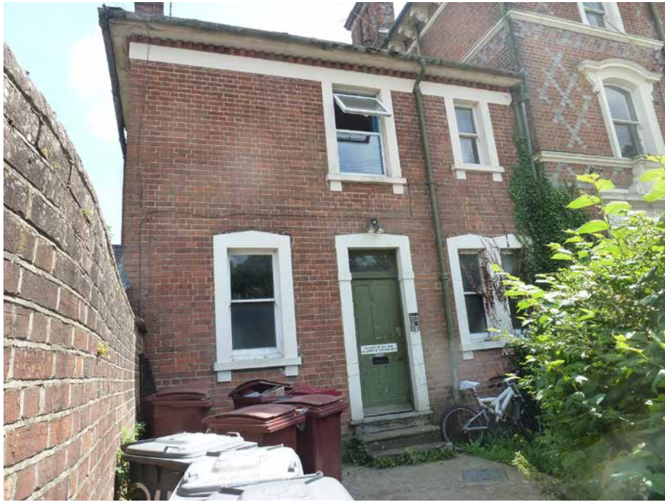
Photo 15: Annex front elevation
