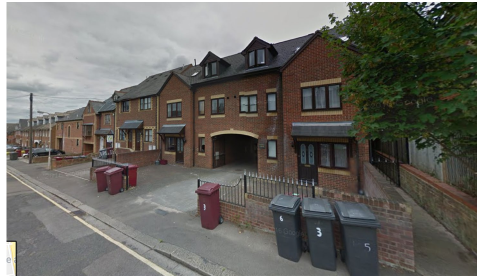
Properties to the East of Franklin Street, modern flatted blocks set back from the street
