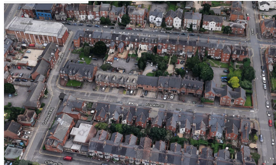
Properties to the East of Franklin Street, modern flatted blocks set back from the street
