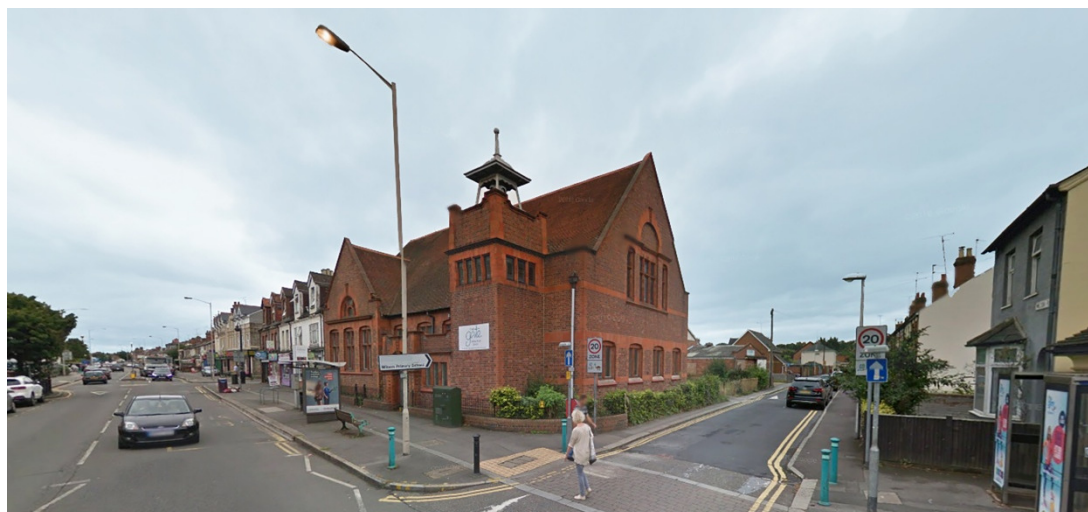
The existing Victorian Chapel at the junction of Oxford Road and Wilson Road
