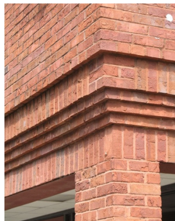
Stepped brickwork as proposed for corner tower
