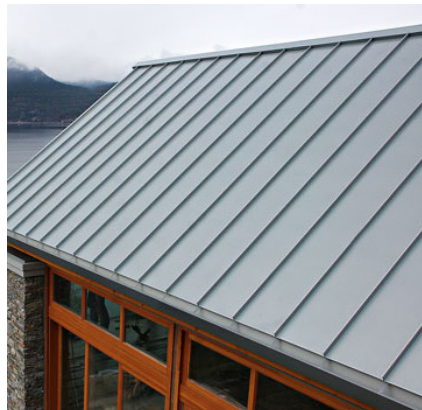
Example of standing seam zinc roof
