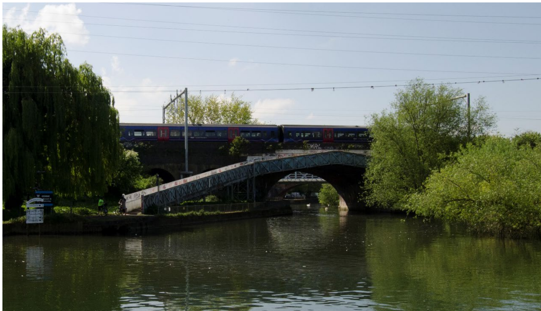
Figure 9.6: Stepped Horseshoe Bridge
