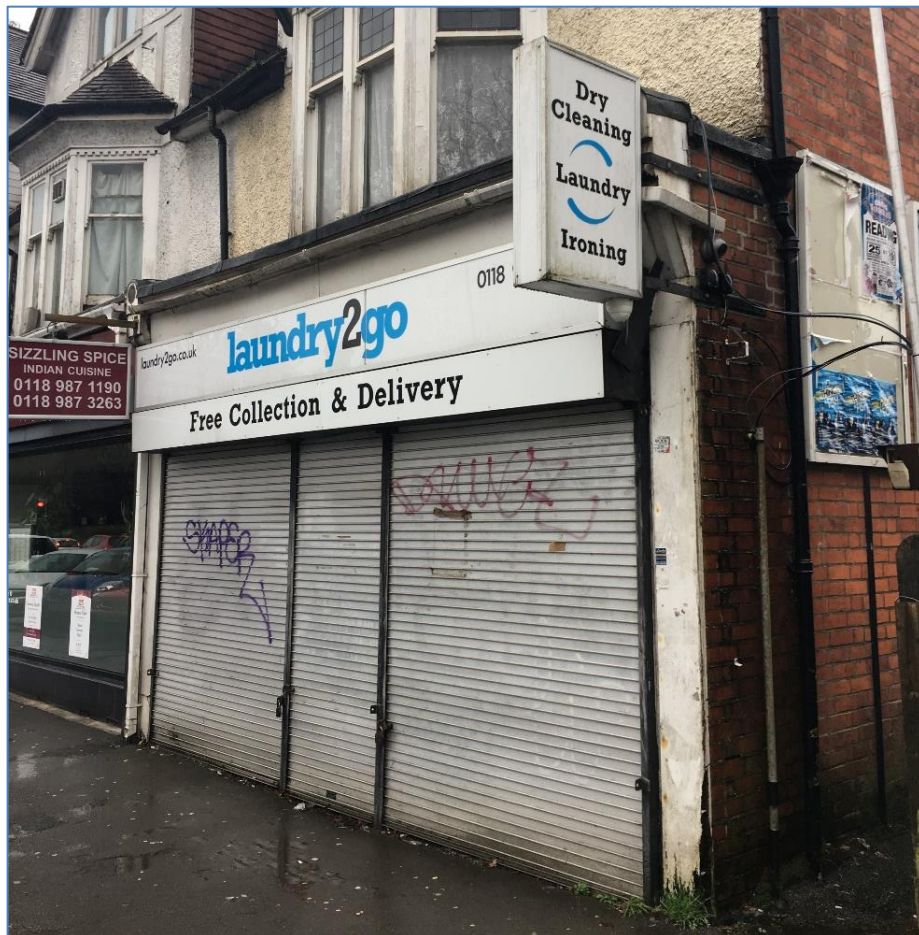
Existing shopfront to be replaced
