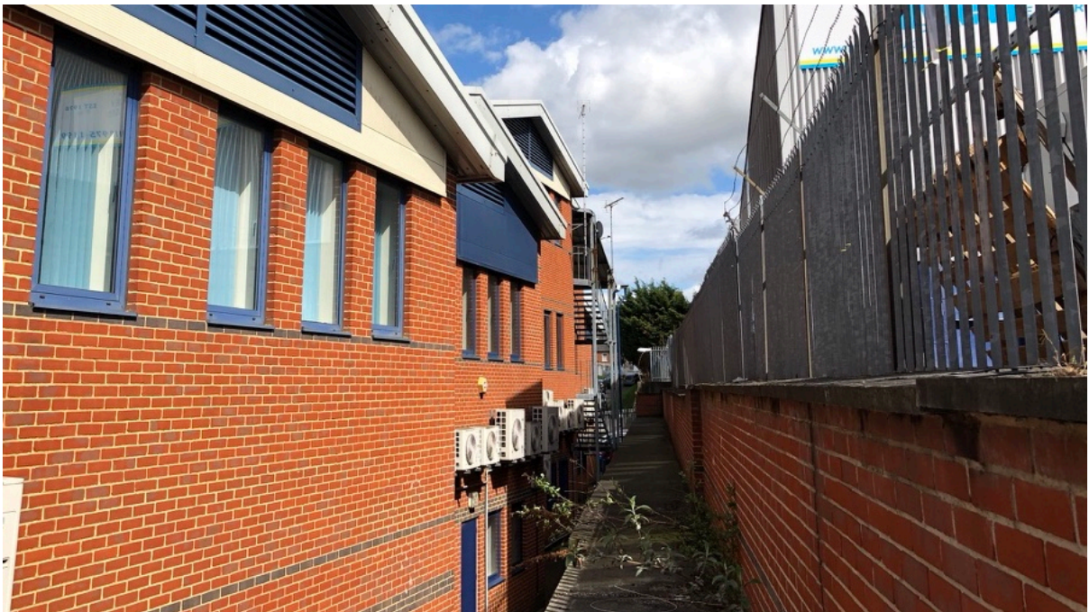
Figure 4 – View of rear of development
