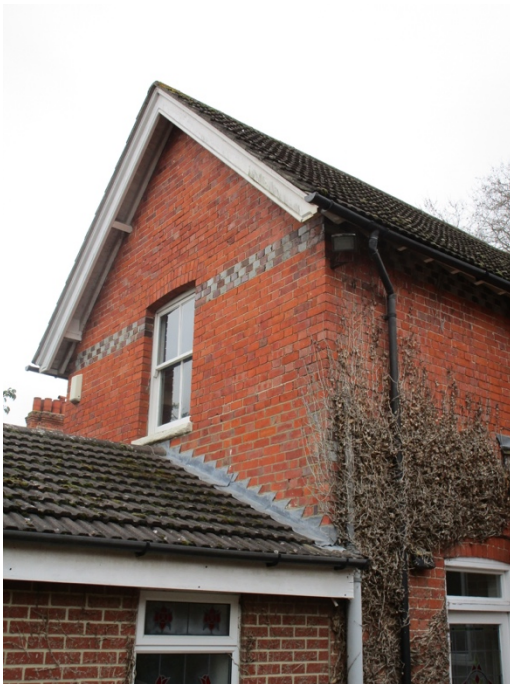
Fig.8 – View of rear of 104 Kendrick Road
