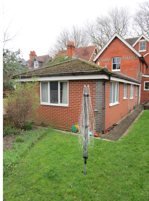
Fig.9 – View of rear of 104 Kendrick Road
