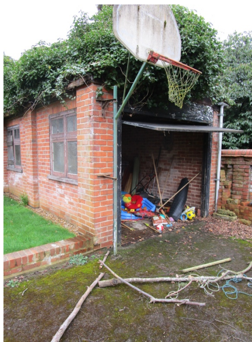
Fig.5 – View of existing garage
