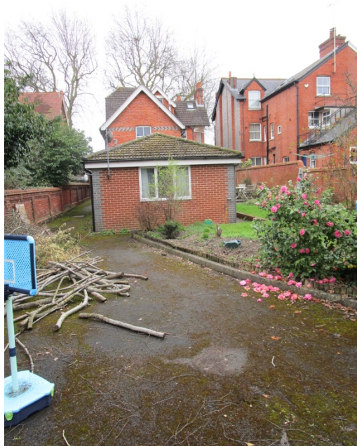
Fig.3 – View of rear of 104 Kendrick Road
