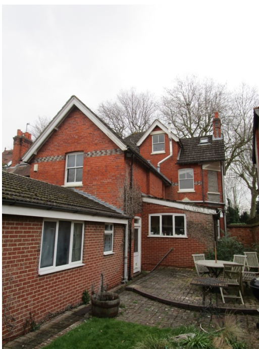
Fig.3 – View of rear of 104 Kendrick Road
