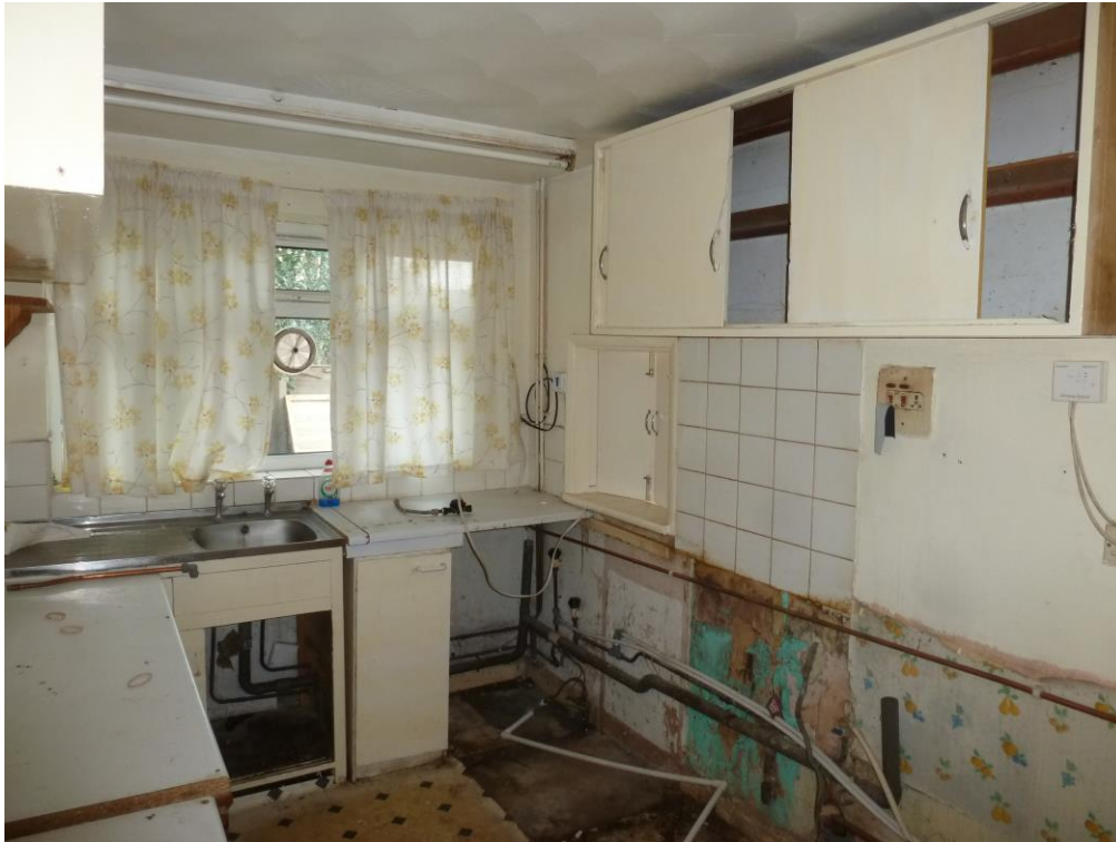
Fig.3: Interior view of existing dilapidated Kitchen
