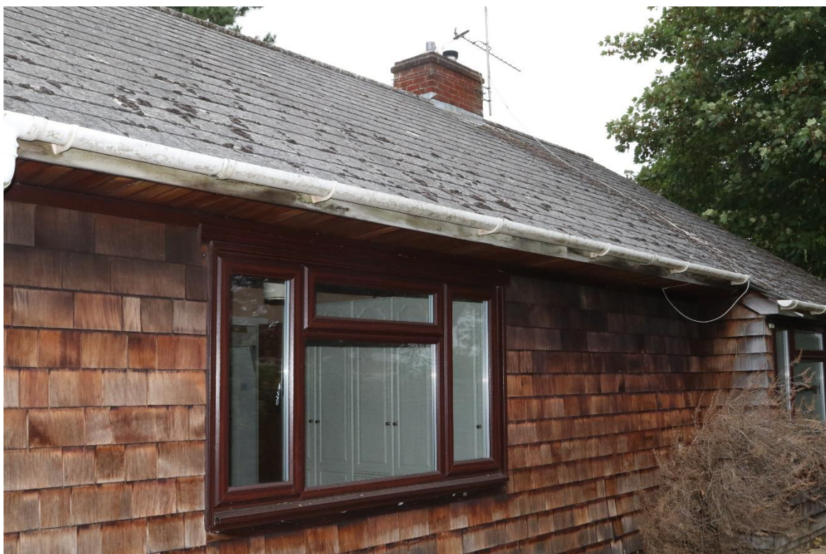
Image 5 – South facing elevation of the building
