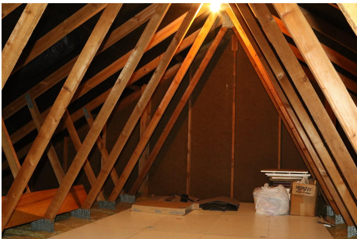
Image 6 – Internal view from within the roof void
