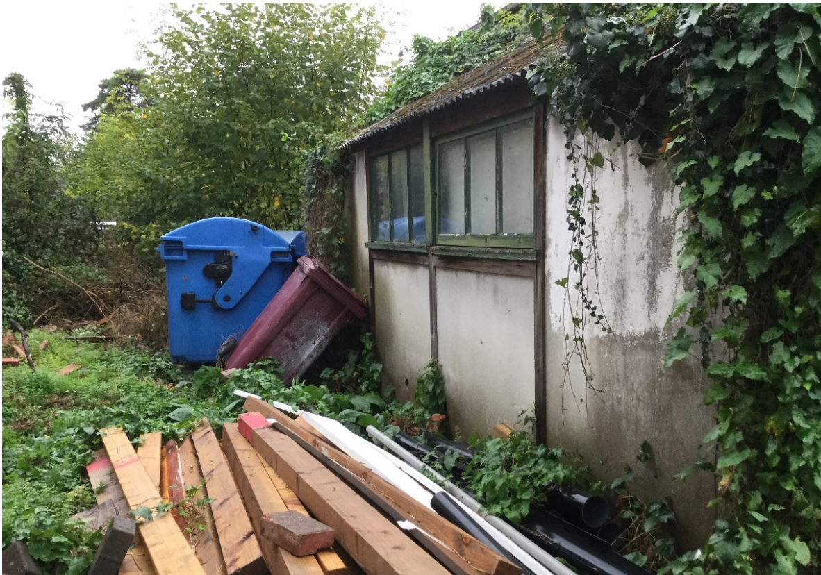
Photograph 2. The south facing elevation of the garage.
