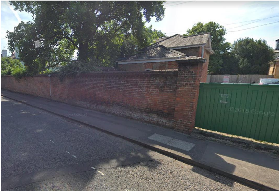
Above: Existing wall along the site boundary on Upper Redlands Road
