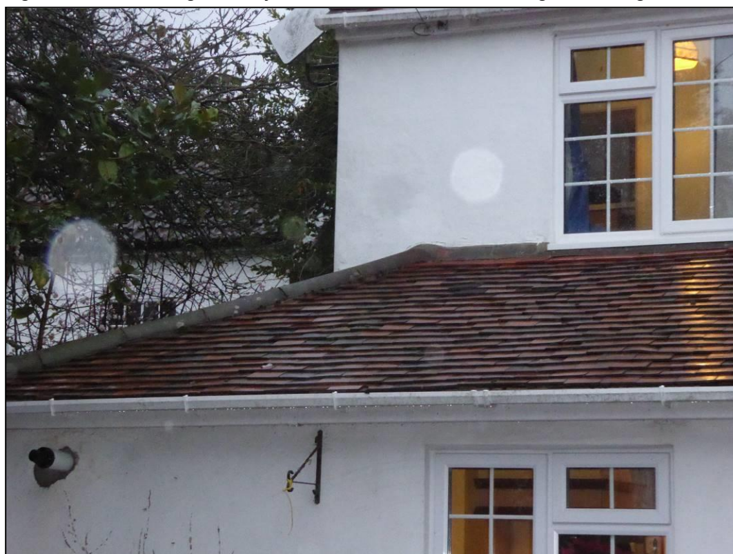
Figure 8. Roof of single-storey extension. Greenwood Cottage, Reading. 05.12.18
