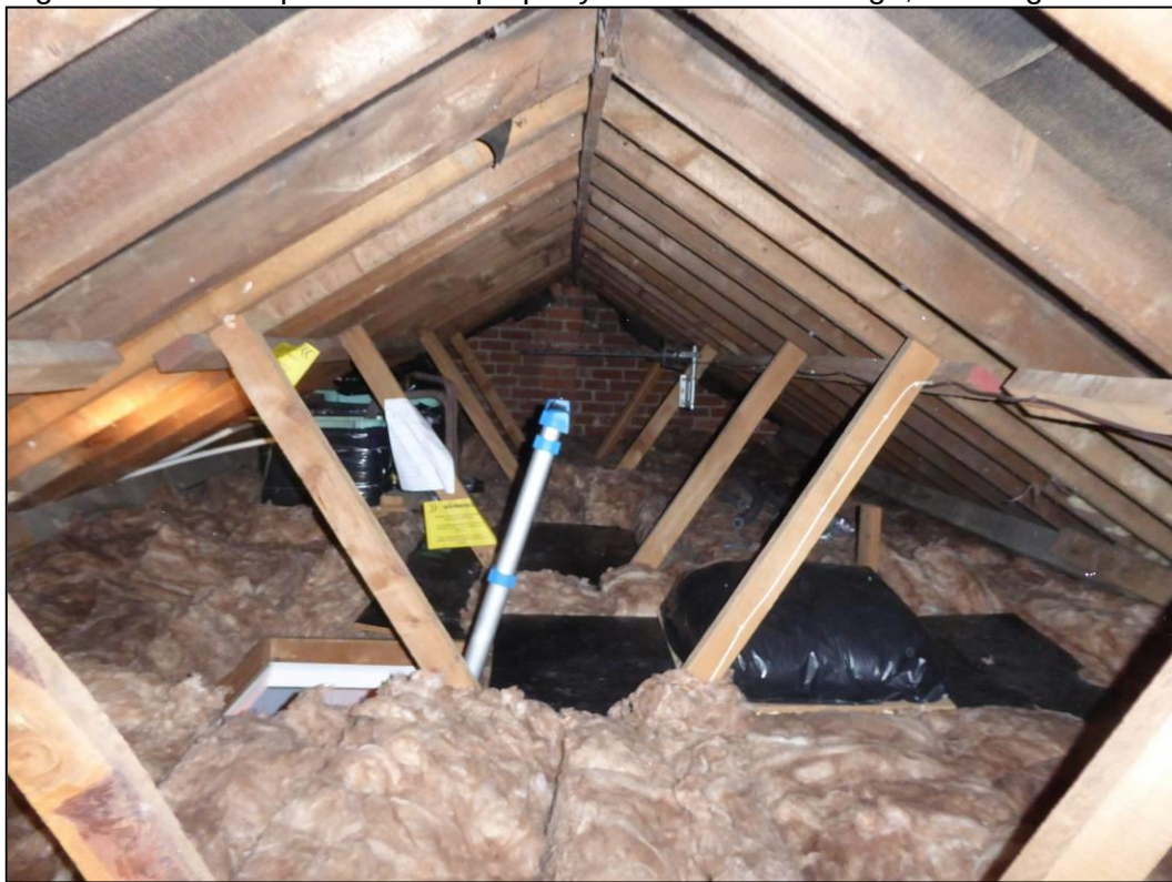
Figure 9. The loft space of main property. Greenwood Cottage, Reading. 05.12.18
