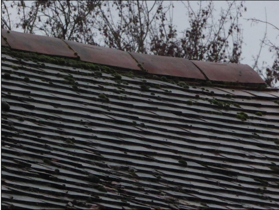
Figure 5. Example of the ridge tiles. Greenwood Cottage, Reading. 05.12.18
