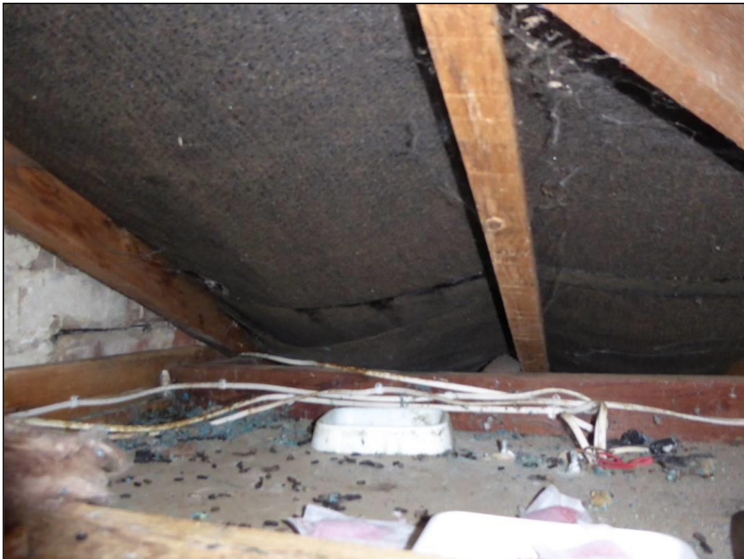
Figure 11. Example of bitumen lining. Greenwood Cottage, Reading. 05.12.18
