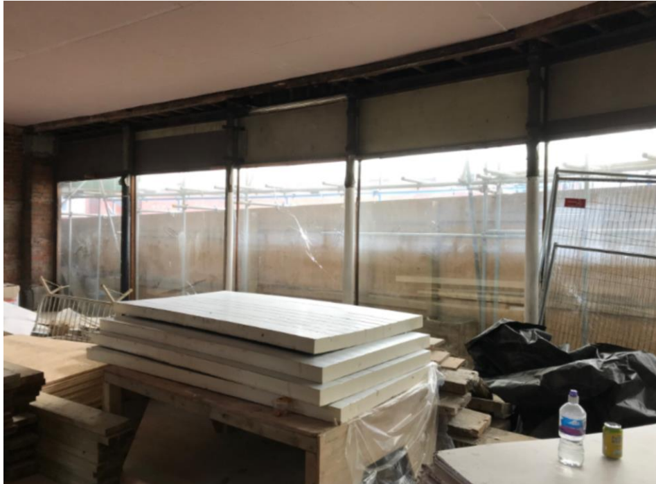
Figure 4: Existing shopfronts to Unit 1, internal view
