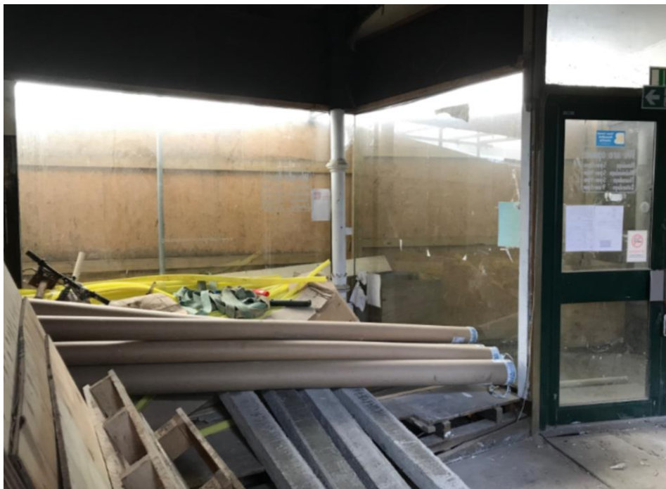
Figure 5: Existing shopfronts to Unit 2, internal view
