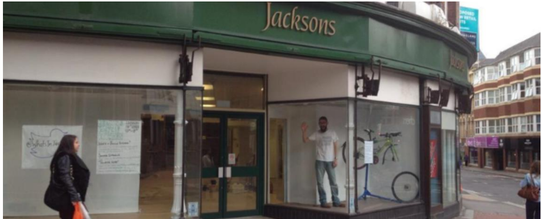
Figure 2: Existing shopfronts to Unit 1, external view
