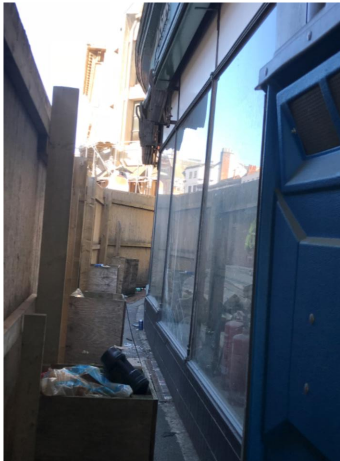
Figure 3: Existing shopfronts to Unit 1, external view
