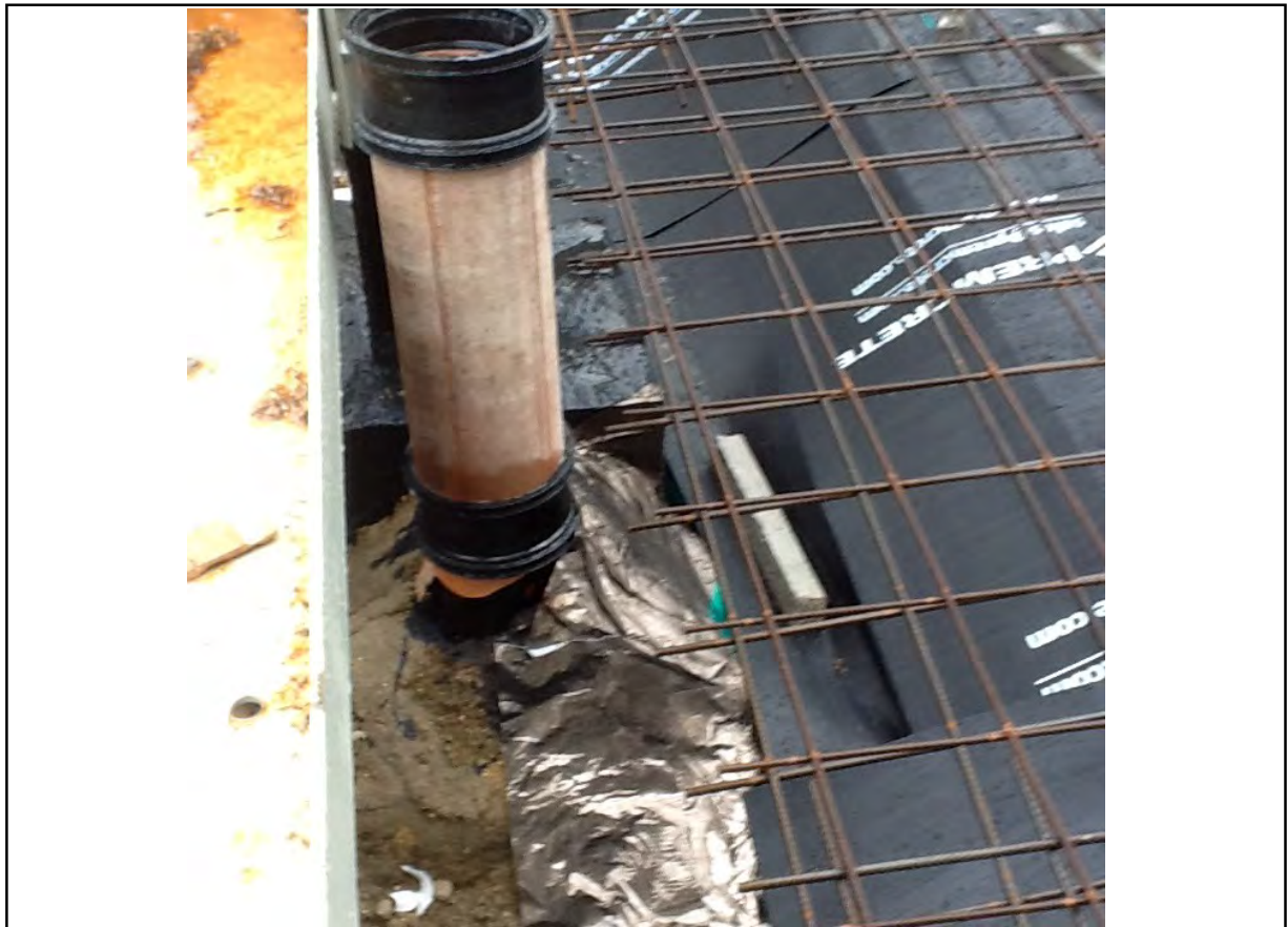
Overview pipe penetration detail
