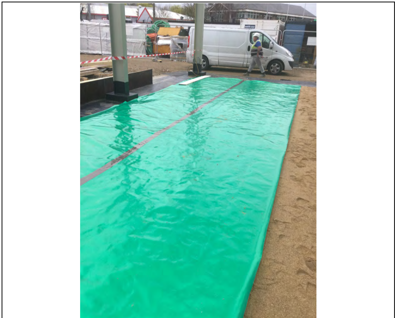
View to A1 corner
