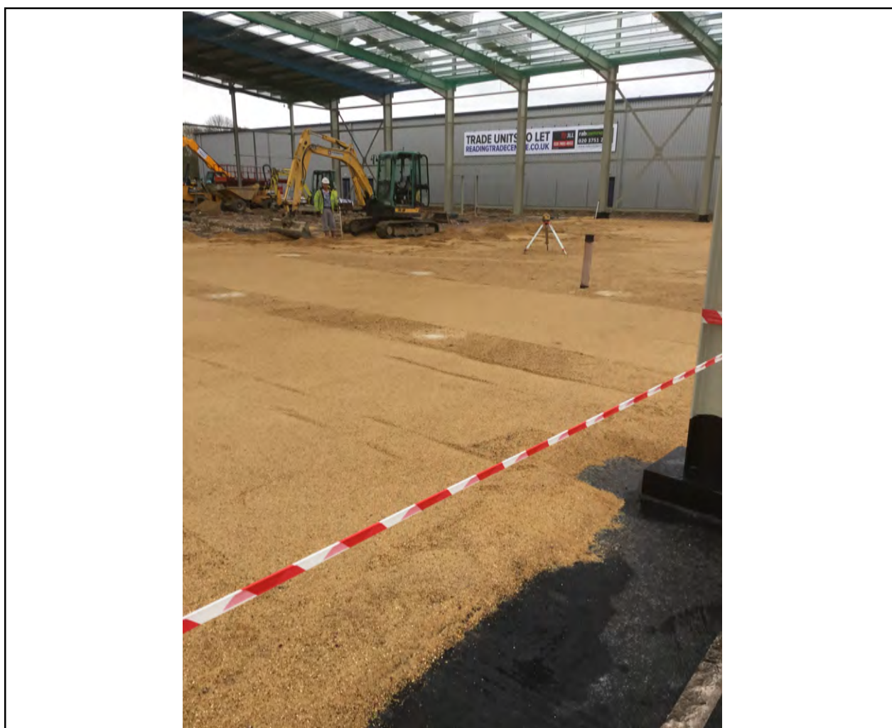
Sand blinding looking to H - 2
