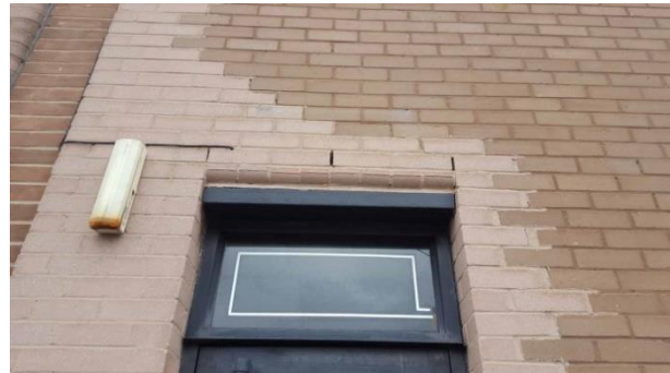
Plate 4.11: Building 2 – Weep Holes
