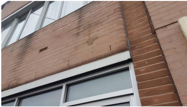
Plate 4.10: Building 2 – Air Vent
