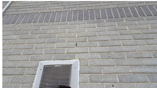
Plate 4.6: Building 1 – Weep Holes
