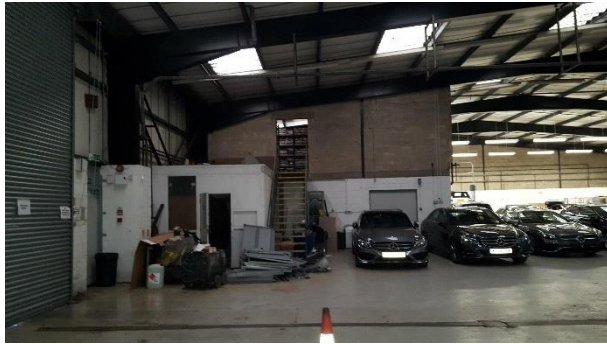
Plate 4.112: Building 2 – Workshop Interior
