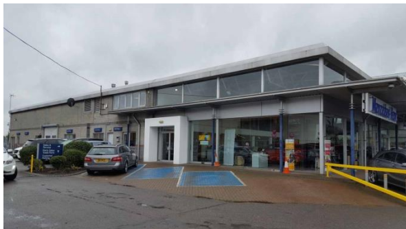
Plate 4.1: Building 1 – Eastern Aspect
