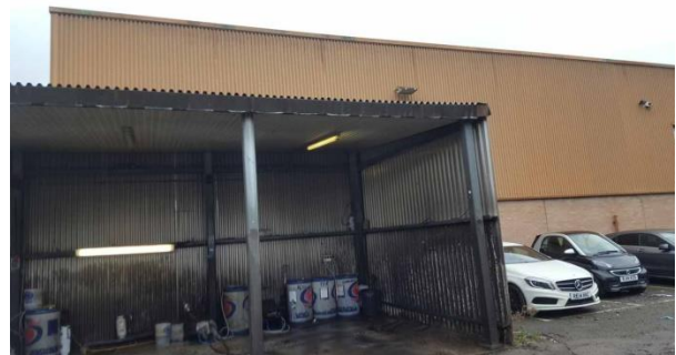
Plate 4.8: Building 2 – Eastern Aspect
