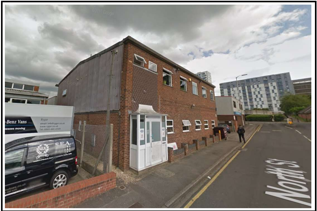
Existing Building from North Street
