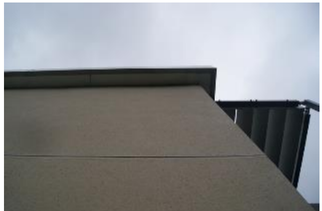
Photograph 10. Concrete rendered walls of new classroom block.
