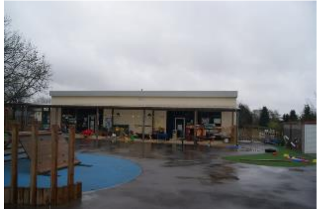
Photograph 8. North-western elevation of the new classroom block.
