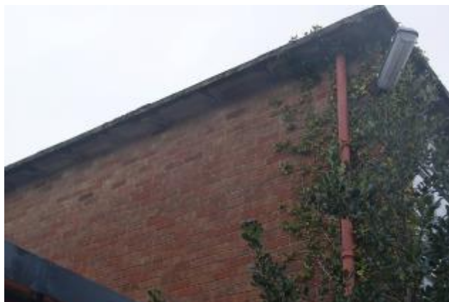
Photograph 4. Eaves of the original school building.
