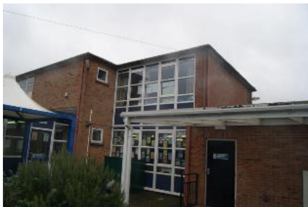
Photograph 3. South-western elevation of the original school building.
