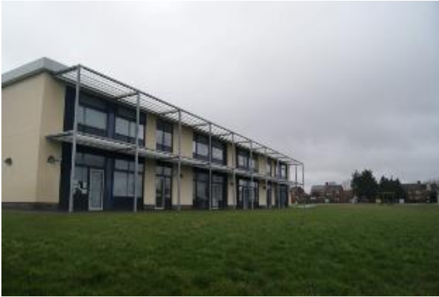
Photograph 7. South-eastern elevation of the new classroom block.
