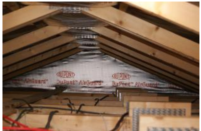
Photograph 12. Roof void in terrapin building.
