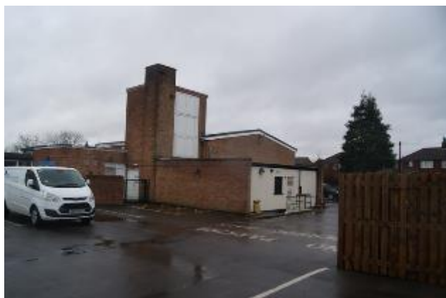
Photograph 1. Eastern elevation of the original school building, showing the tower section (location of loft void).
