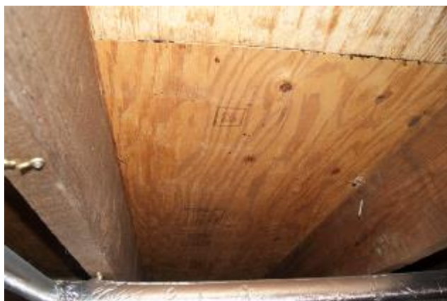
Photograph 6. Underside of roof in tower section loft void.
