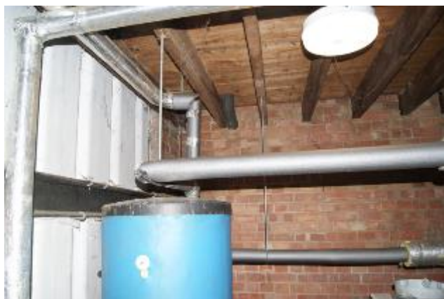
Photograph 5. Loft void in tower section of the original school building (first level).
