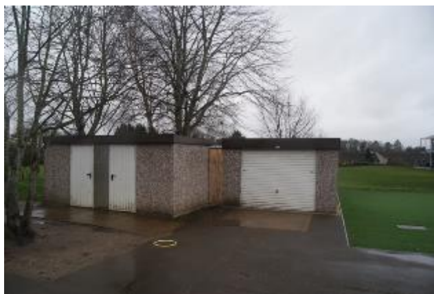
Photograph 13. Two precast storage buildings located to the west of the terrapin buildings.
