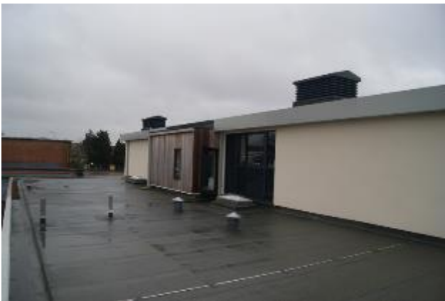
Photograph 9. Flat roof of new classroom block.
