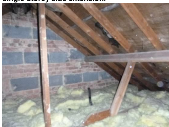
10. internal view of the roof space.
