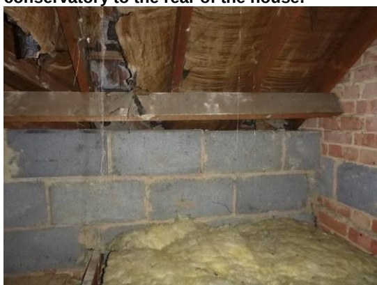
11. Blockwork wall along the front of the roof space.
