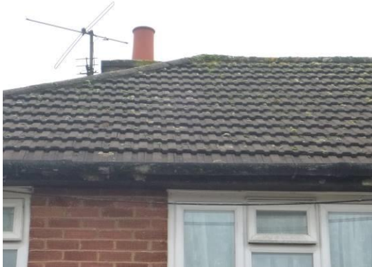
3. Interlocking roof tiles in place and tightly fitted.
