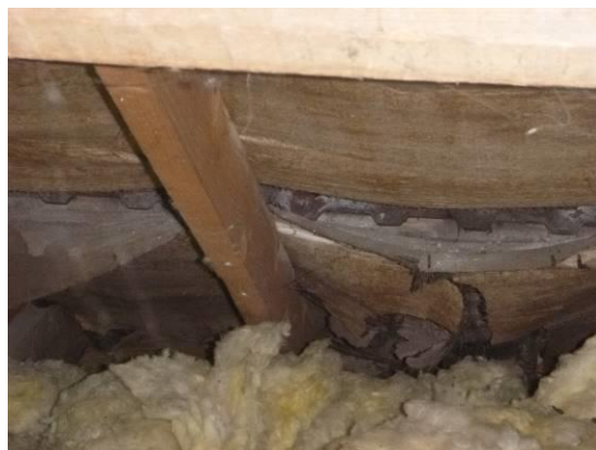
14. The eaves mostly filled with fibreglass insulation.
