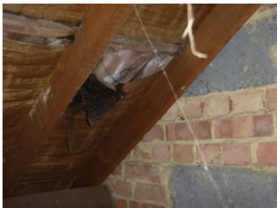
15. The brick and blockwork party wall.
