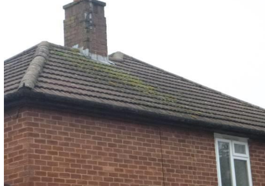
6. Lead flashing tightly fitted around the chimney.
