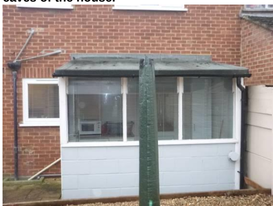
9. The bitumen roofing felt tightly fitted on the conservatory to the rear of the house.
