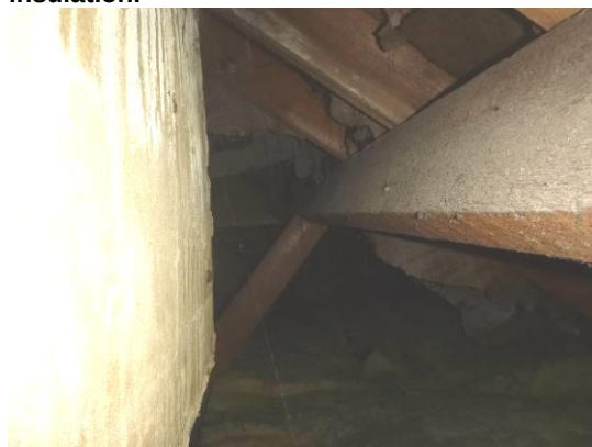
16. The rendered chimney and roof space visible beyond.
