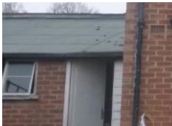
8. The bitumen roofing felt tightly fitted on the single-storey side extension.
