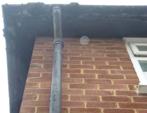
7. Timber soffits tightly fitted around the eaves of the house.
