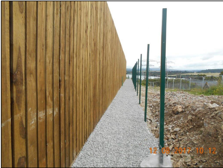
Figure 10 Illustration of acoustic barrier
