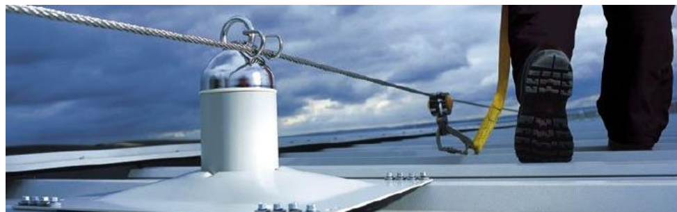
Figure 8: Work restraint safety wire system
