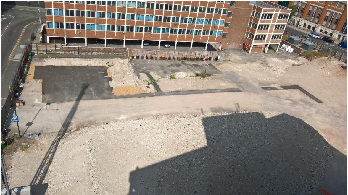
Plate 2 – Compound area located between Garrard Street and Station Hill with crushed aggregate stockpiles where Western Tower was previously demolished.
