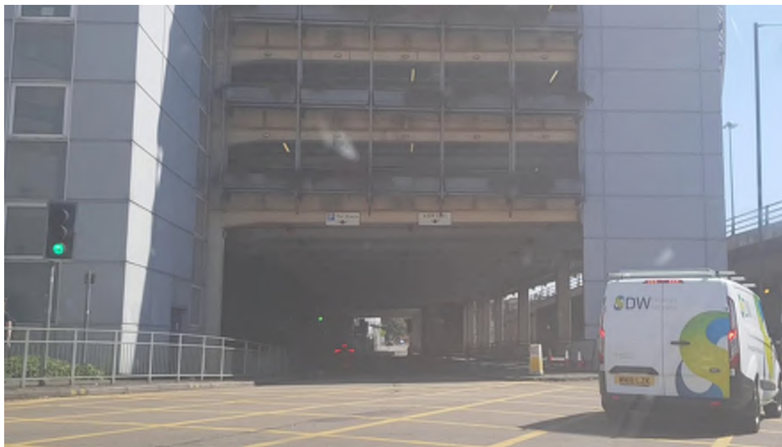
Lane guidance signs to The Oracle (Riverside) Car park Entrance and A329
