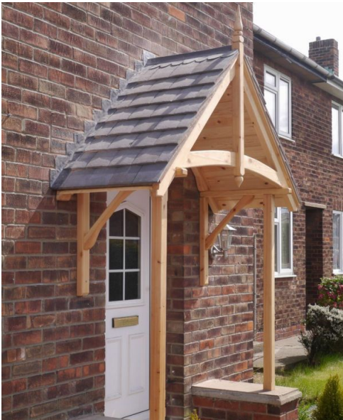
Apex timber pitched awning
