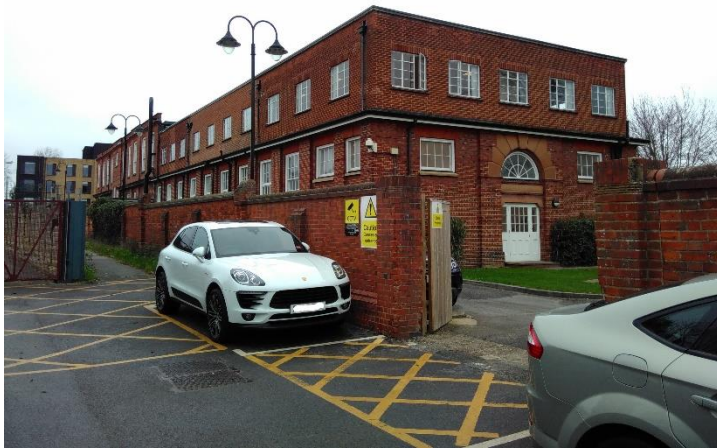
Building LO22, looking north-west from Acacia Road.
