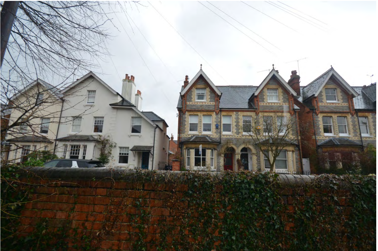
Plate 21: Looking south towards the buildings on the opposite side of New Road
