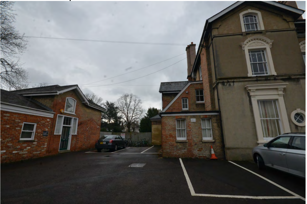
Plate 5: The development area viewed between existing buildings on Upper Redlands Road
