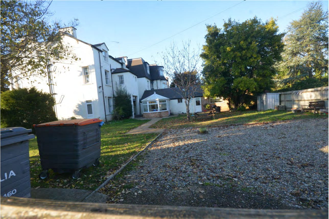
Plate 12 The Side elevation of 19 Redlands Road
