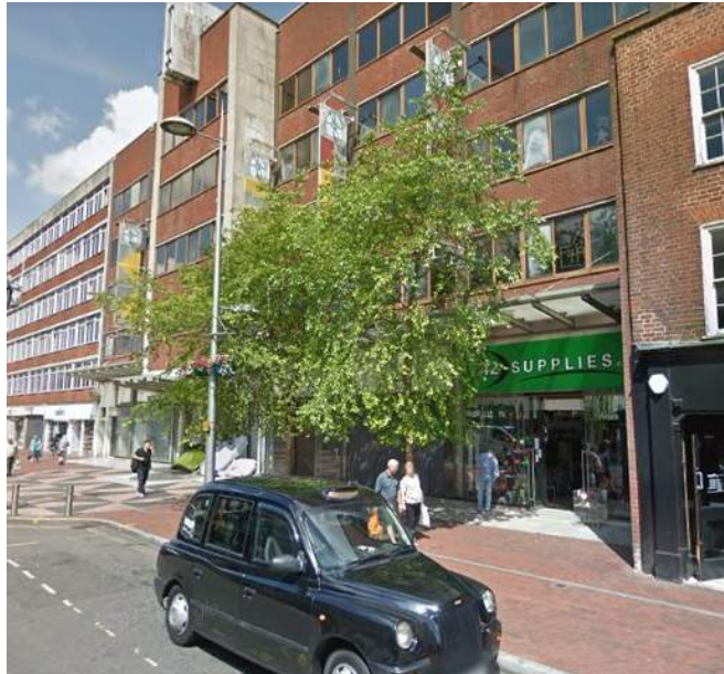
The trees that we will protect from the adjacent works
