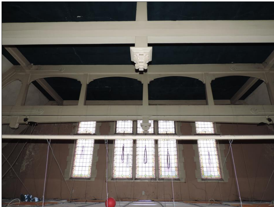
Photo 10 Restricted view of original timber frame roof structure, now concealed by 20 th century suspended ceiling.
