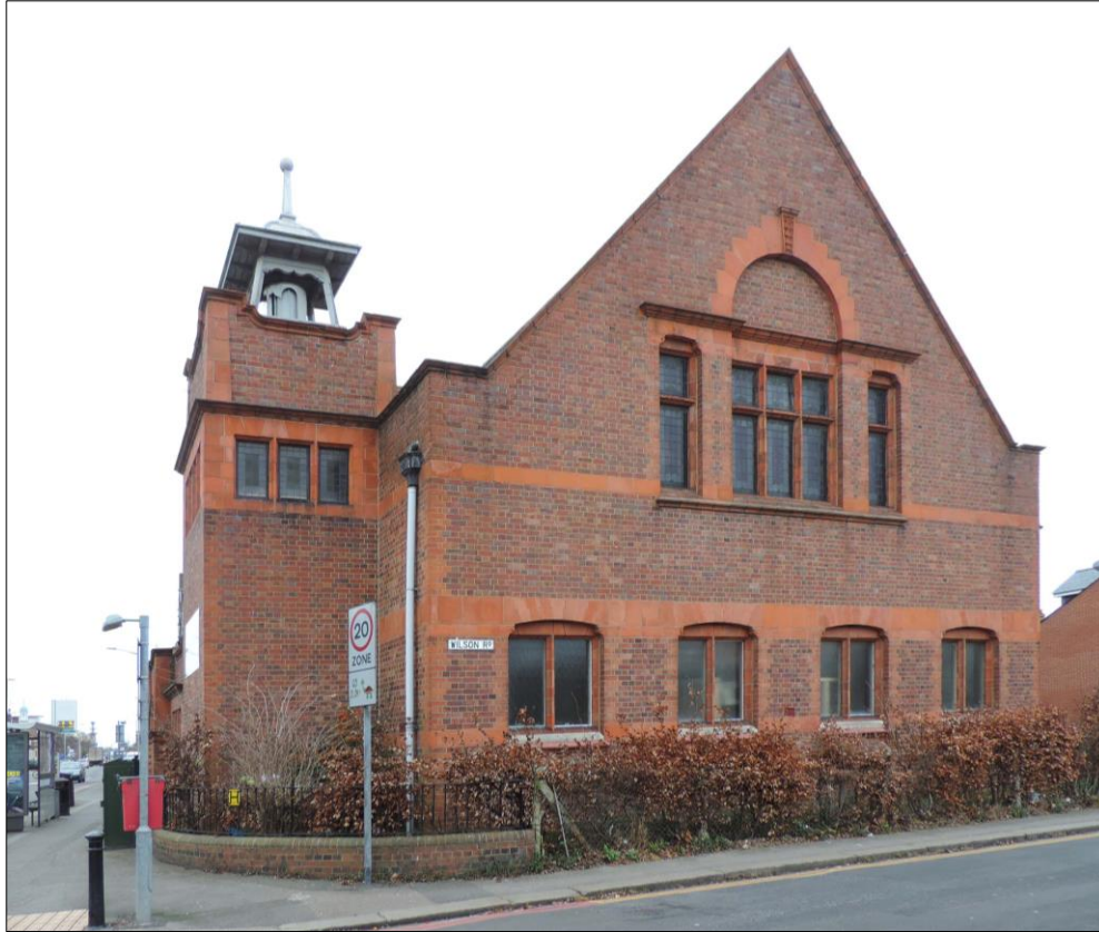
Photo 3 Southeast facing view of west gable.
