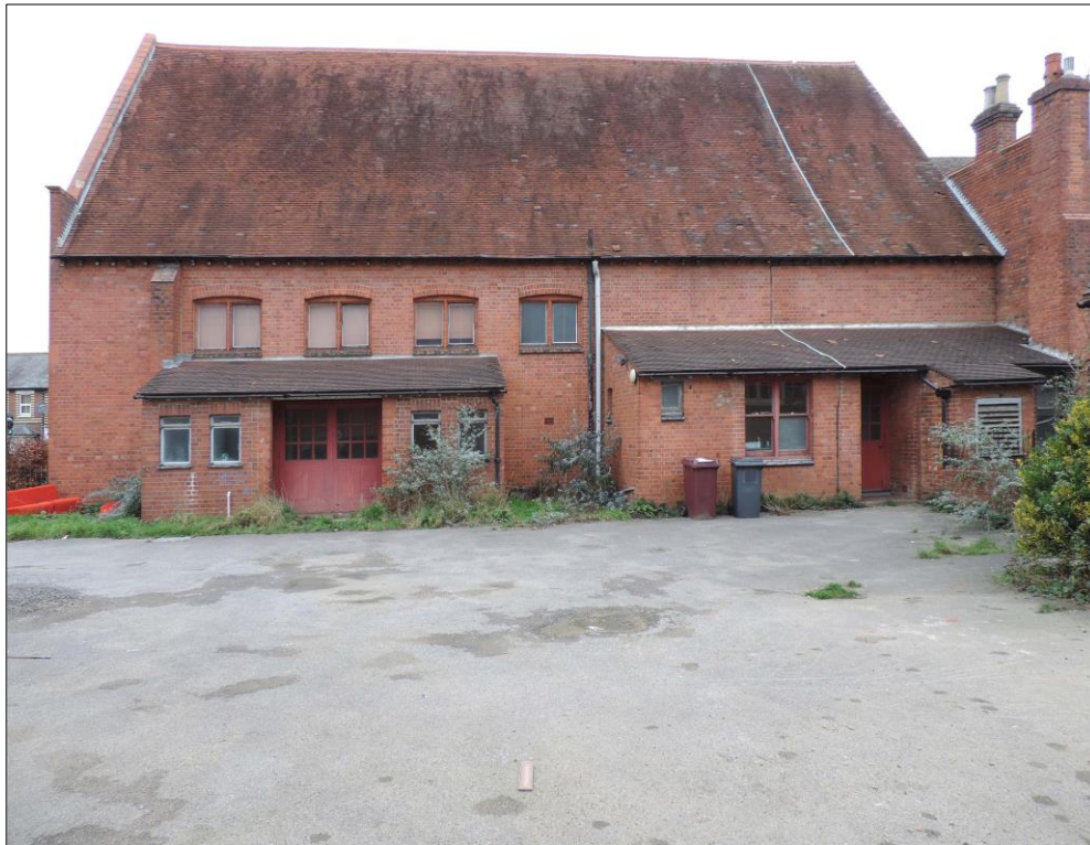
Photo 4 Northeast facing view of rear elevation (south).
