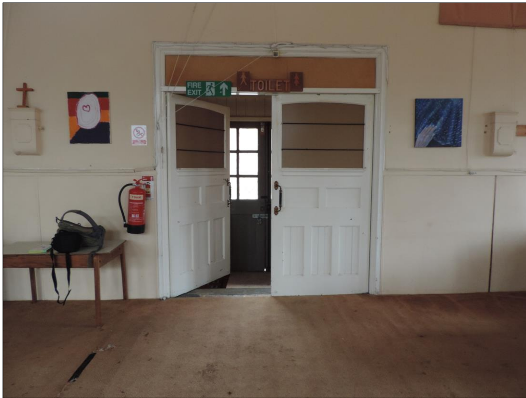
Photo 5 Southwest facing view of double doors within southern wall.
