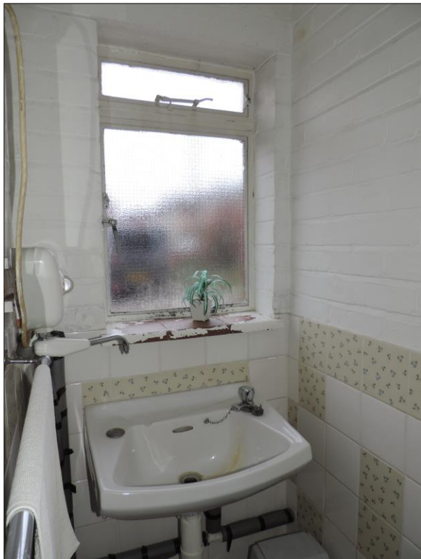
Photo 7 Southwest facing view of washbasin housed in the lean-to to the southwest of Grovelands Church.
