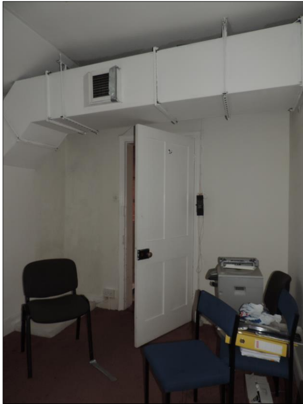
Photo 6 Southwest facing view from interior of small meeting room / office housed in the lean-to to the southeast of Grovelands Church.
