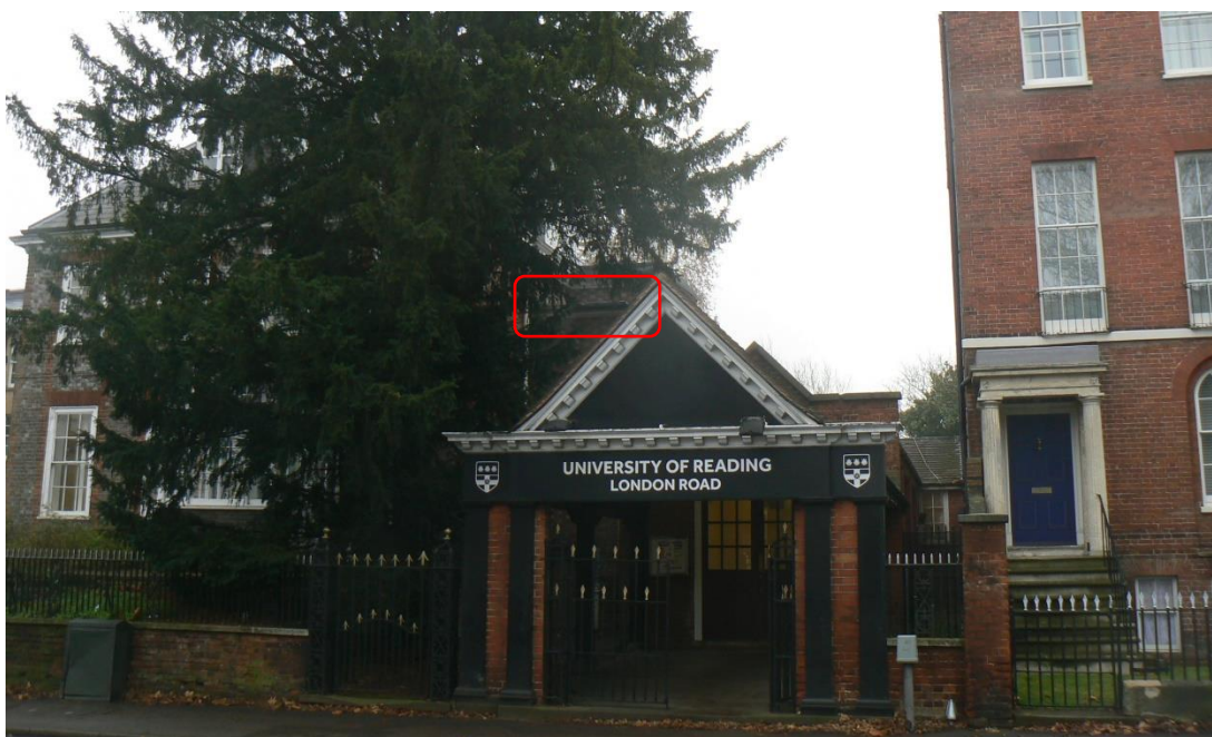
Figure 2: The subject roof is outlined in red
