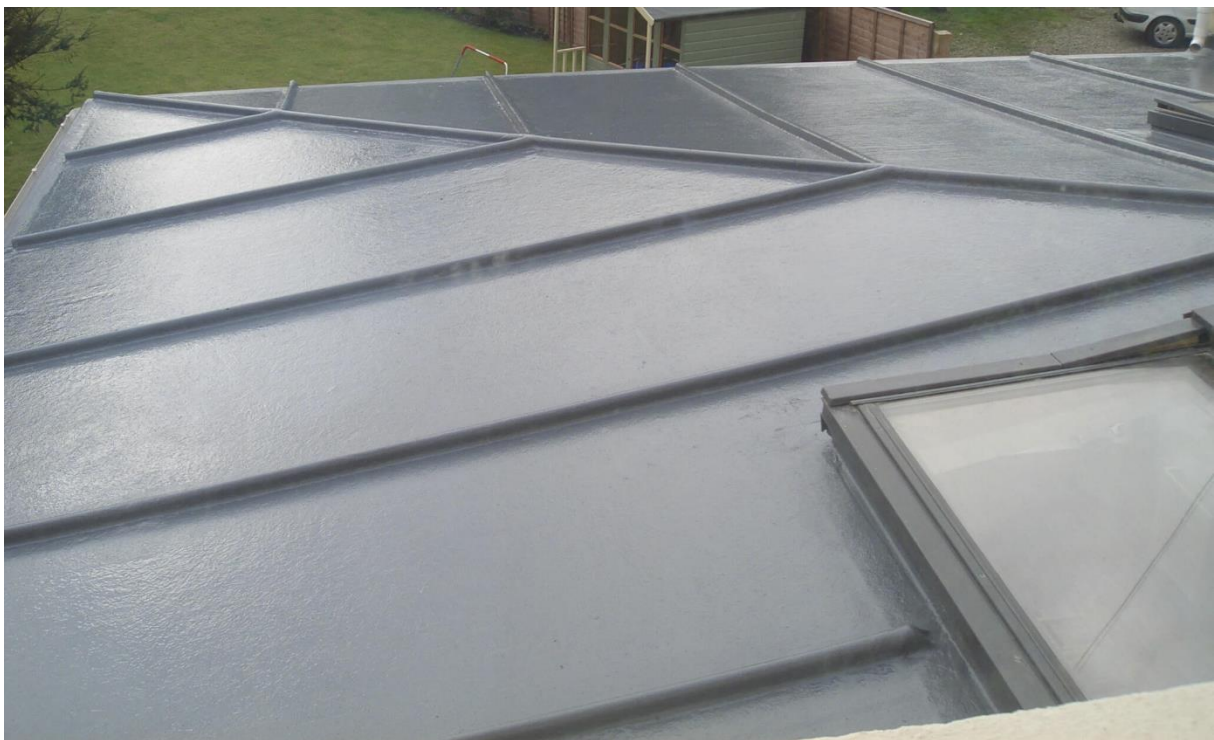
Figure 4: A typical application of lead grey liquid applied polymer.
