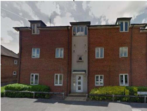
3 Storey Apartments - South along Silver St
