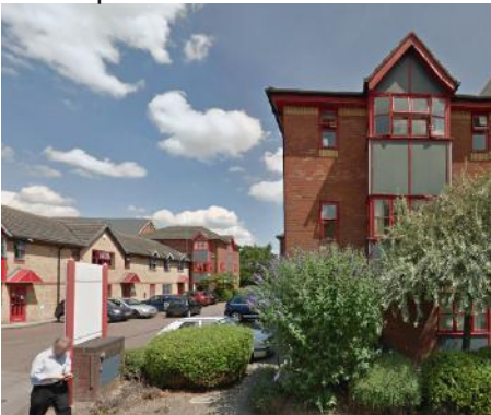
3 Storey Windsor Court - adjacent to the site
