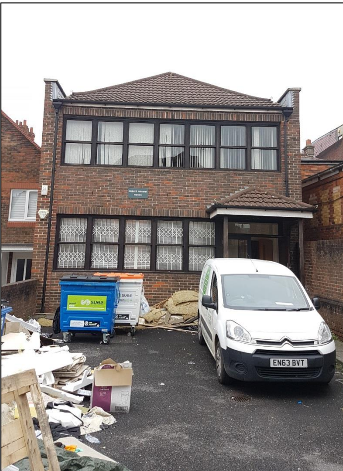
Plate 2. Building 1b (exterior) (View: east)
